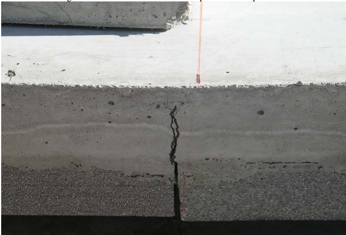
Figure 11: Flexural failure of the 20 ft long panel due to overloading
