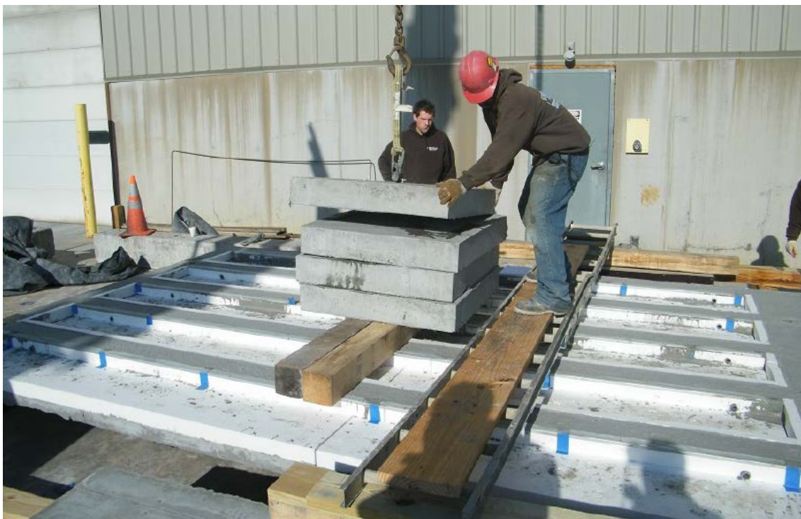
Figure 8: Loading the 16 ft long on the stud side (16 ft long panel)
