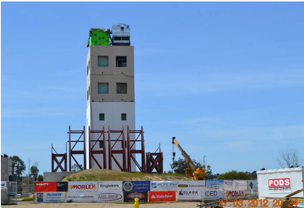
Figure 1. Five-Story Concrete Frame Test Specimen.
