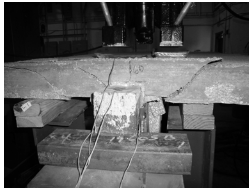
Fig. 8 Hanger Punched Through Slab
