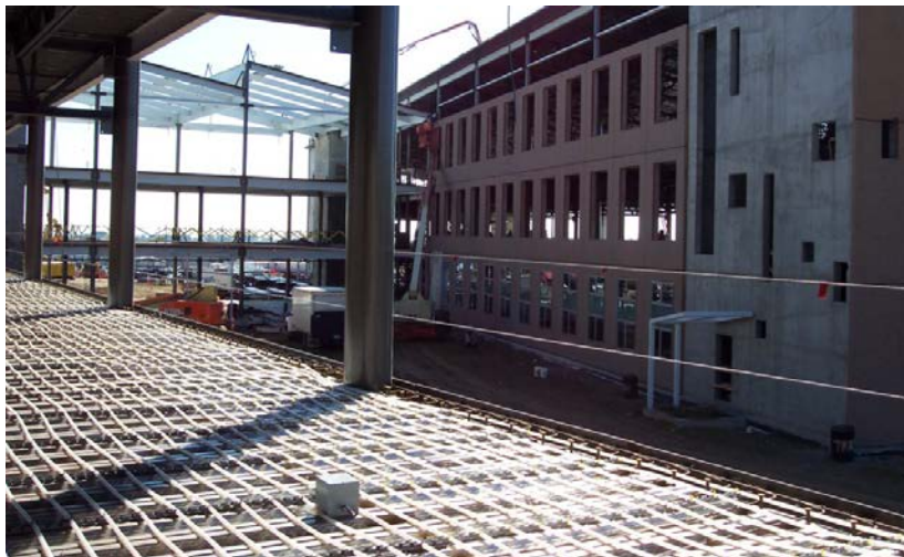
Fig. 4 Radiant ceiling cooling systems helped the National Renewable Energy Lab's Research Support Facility reach their goal of LEED Platinum and Net Zero.
