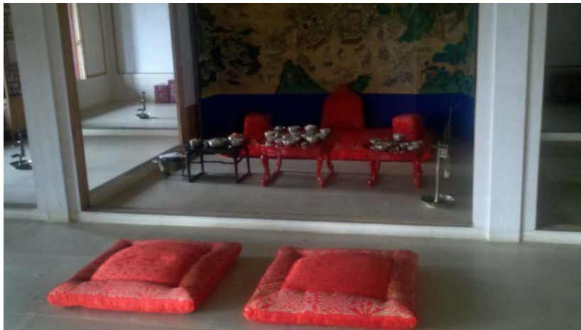
Fig. 2 Under-floor heating systems were efficient and effective.
