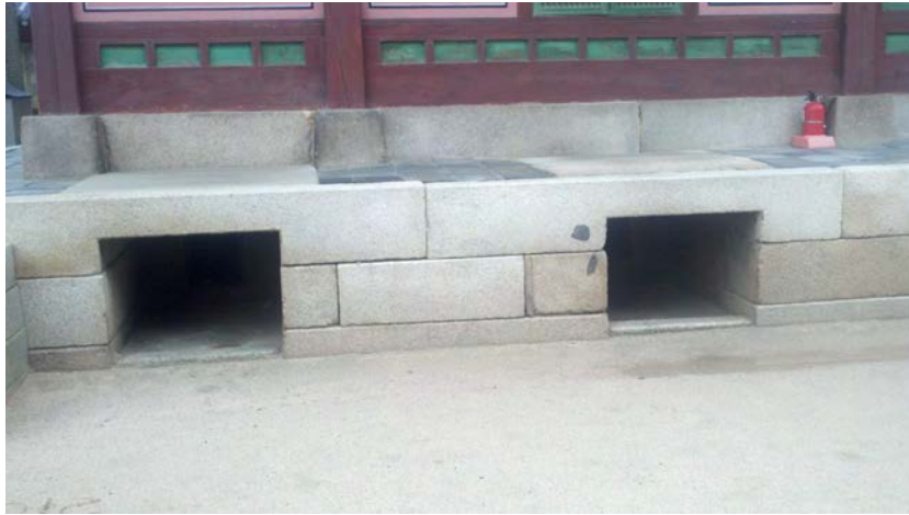
Fig.1 Hot smoke from ovens such as these at the Gyeongbokgung Royal Palace in Seoul, South Korea was drafted through under-floor trenches, creating warm living spaces.
