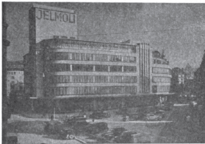
Fig. 3 Jemoli Department Store in Switzerland is reportedly the first large-scale commercial building to utilize radiant cooling. 3
