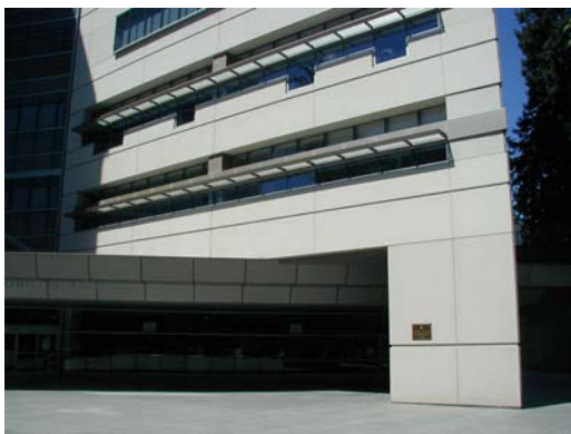
Figure 1. Example of Cladding Panels Mounted on King Library at San Jose State University.
