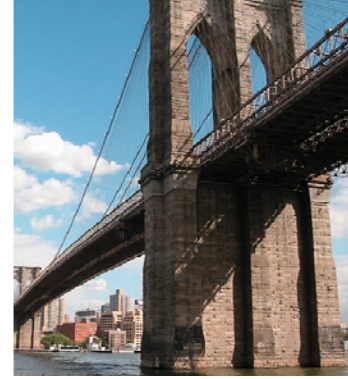
Brooklyn Bridge Abutment
