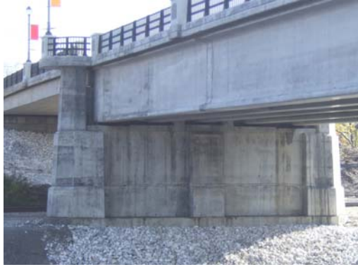
Cross Street Bridge Abutment
