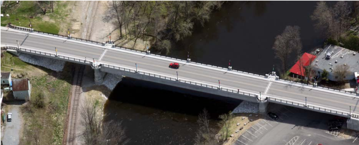
The Completed Cross Street Bridge
