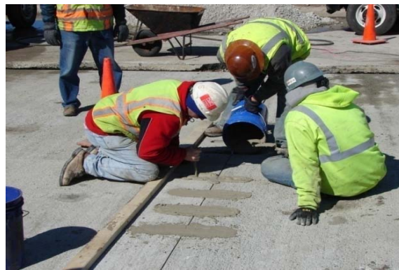
Fig. 3 A variation for Installing Dowel Bars Using the DBR Method
