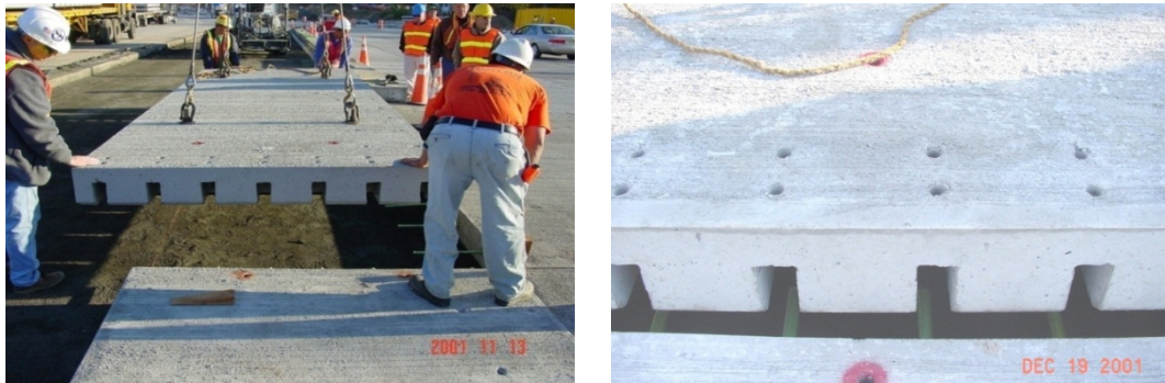
Fig. 5 A Scheme for Providing Load Transfer in JPrCP.
