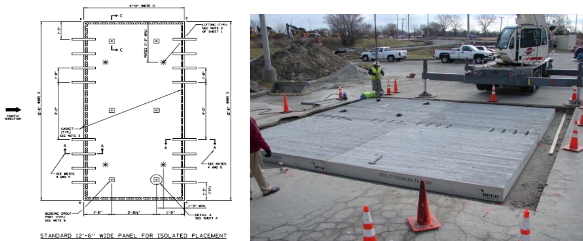
Fig. 12 Illinois Tollway Intermittent Repair System.
