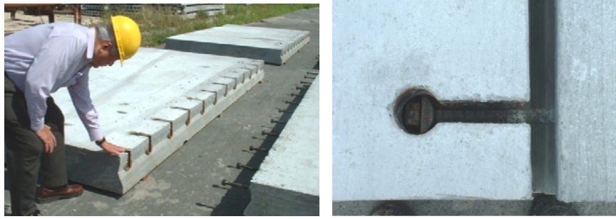
Fig. 11. The Kwik Slab Joint Interlocking System.
