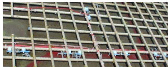
Fig. 4. Electrical and vibrating wire strain gauge installation in panel P2
