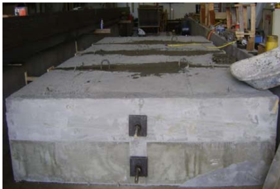
Fig. 9: Specimen after Grouting Shear Keys
