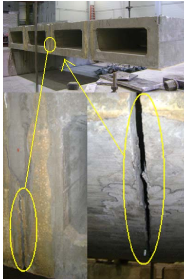
Fig. 20 Side (Bottom Left) and Underside (Bottom Right) Cracking at Interior Joint
