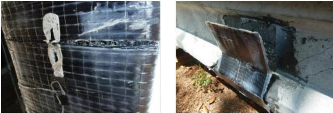
Fig. 11: (left) Rupture of longitudinal CFRP; (right) Debonding of CFRP U-wrapping
