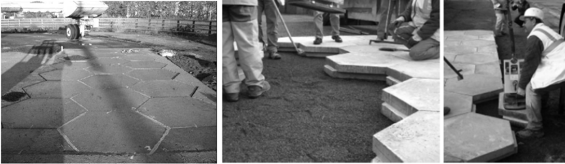
Fig. 1 Installation of Keyed Hexagonal Slabs
