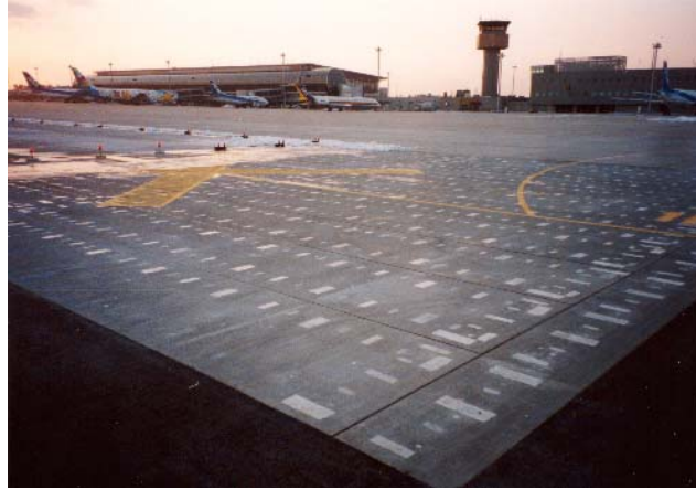
Fig. 12 Constructed PCP at Sendai Airport
