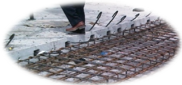
Fig. 6 Use of Cast-in-place Reinforced Gap Slabs
