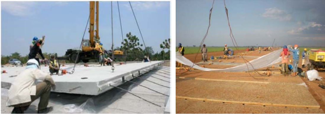
Fig. 4 Indonesia PPCP Installation
