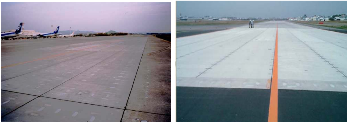
Fig. 9 Airport Applications (Osaka Airport, 1998; Fukuoka Airport, 2003)
