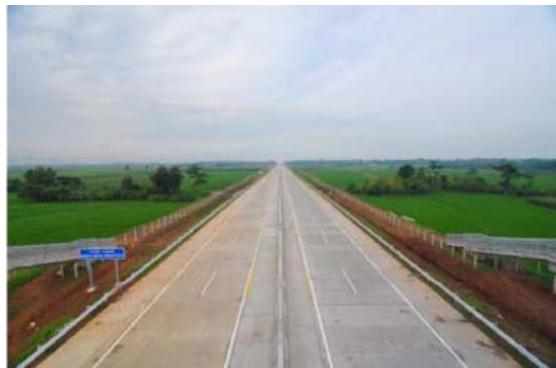
Fig. 5 View of the Completed PPCP Project
