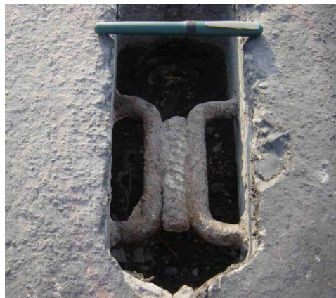
Fig. 19 Welded Lift Loop Connection
