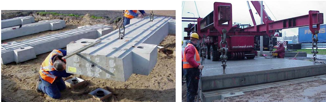
Fig. 16 ModieSlab Installation
