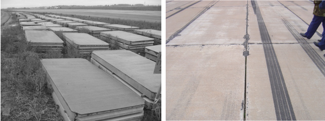
Fig. 18 Soviet Era Precast Panels – Storage and an Installed Site
