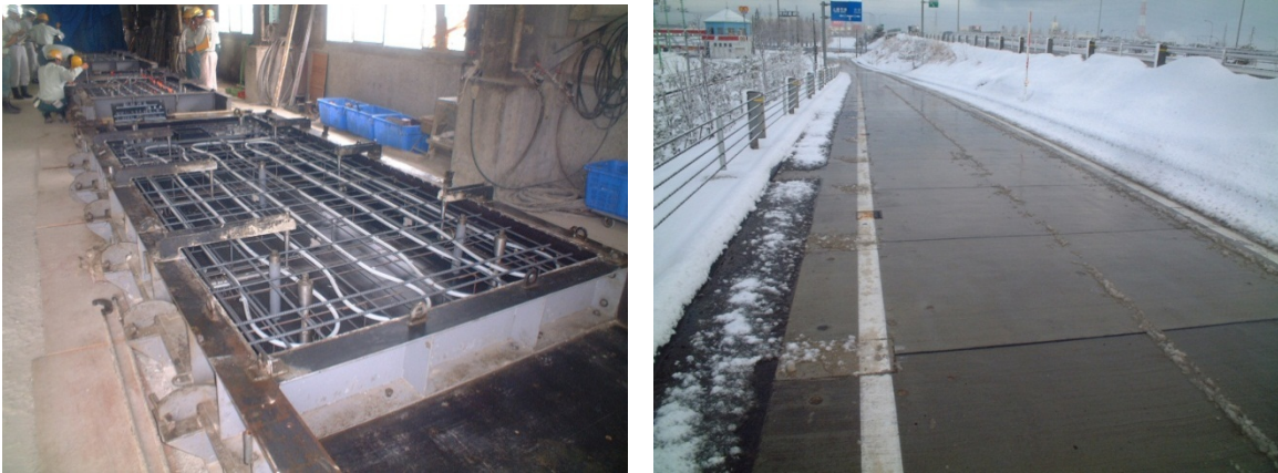
Fig. 13 Heated Precast Panel Fabrication and Installed Project
