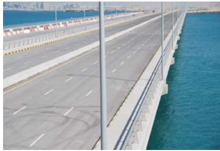
(a) Main Highway Bridge
