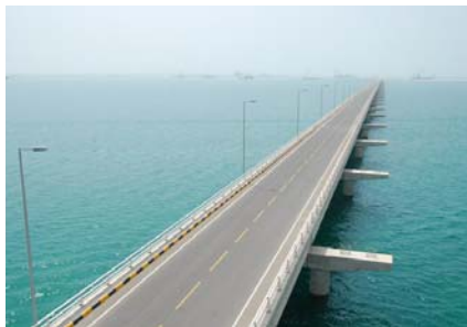
(c) Trestle Bridge
