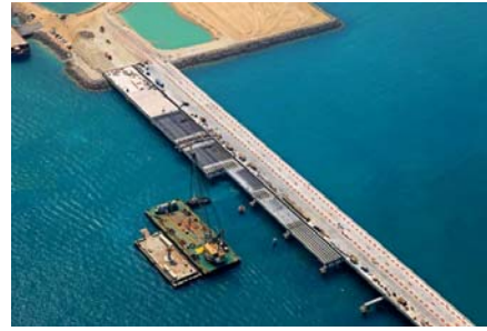
(b) Utility Bridge
