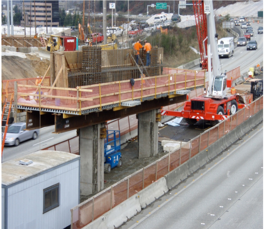
Figure 3 - Pier 3 Construction in I-405 Median
