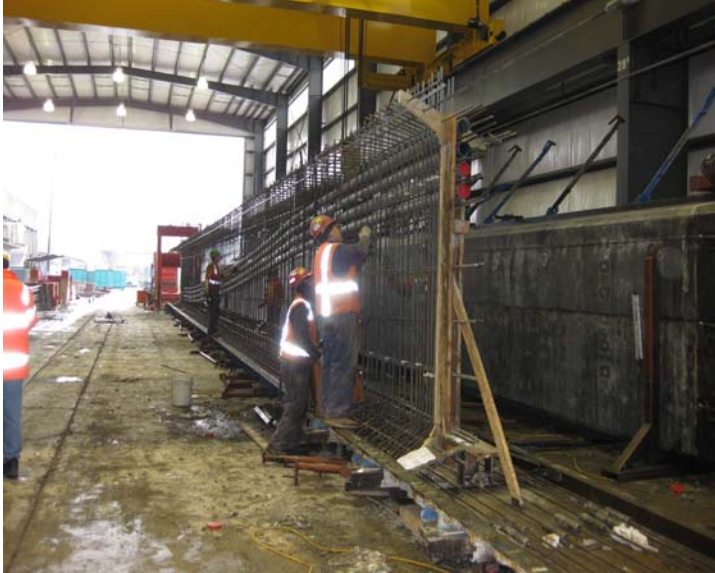
Figure 8 - Girders Being Fabricated at Precast Plant
