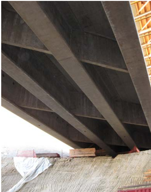
Figure 12 - Typical Intermediate Diaphragms
