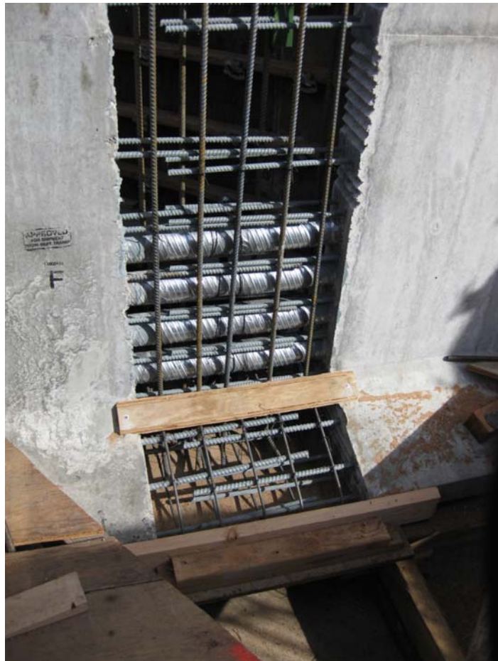
Figure 11 - Girder Splice Region Prior to Concrete Placement
