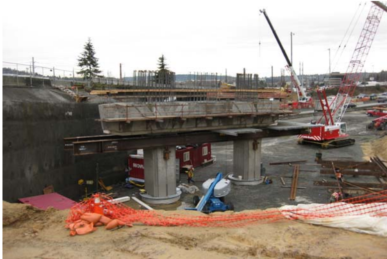
Figure 7 - Pier 2 with Isolation Casings
