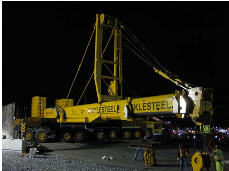
Figure 10 - Sicklesteel 650 Ton Crane
