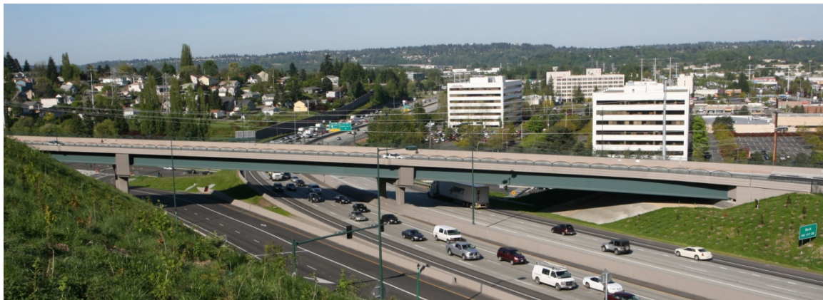
Figure 1 - View of Existing and Completed Benson Road Bridge
