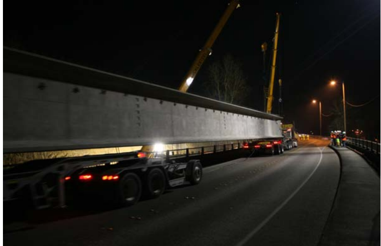
Figure 9 - Girders Being Trucked to Site
