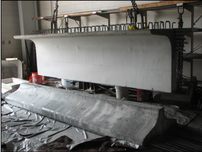
Figure 1. Bottom flange completely cut from the specimen (Girder 1)
