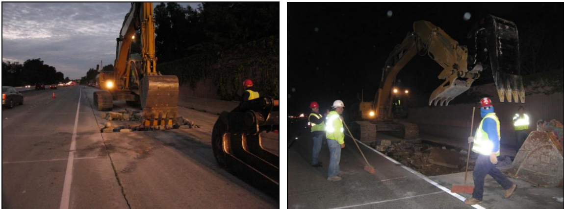
Figure 7 – Demolition of distressed pavement and underlying base
