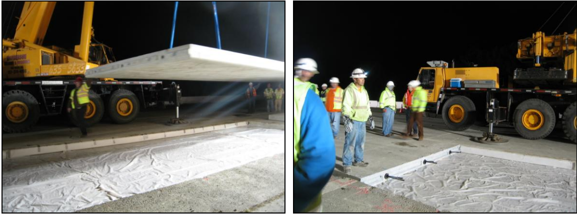
Figure 11 – Installation of PPCP panels
