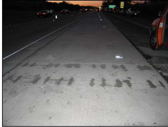
Figure 14 (continued) – (c) completed installation
