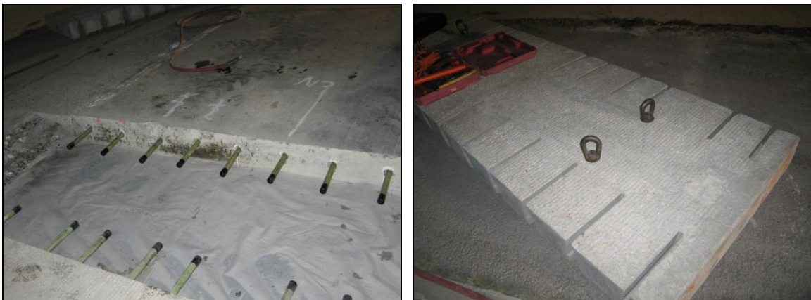
Figure 14 – (a) Dowels installed in existing pavement; (b) permanent drop-in panel
