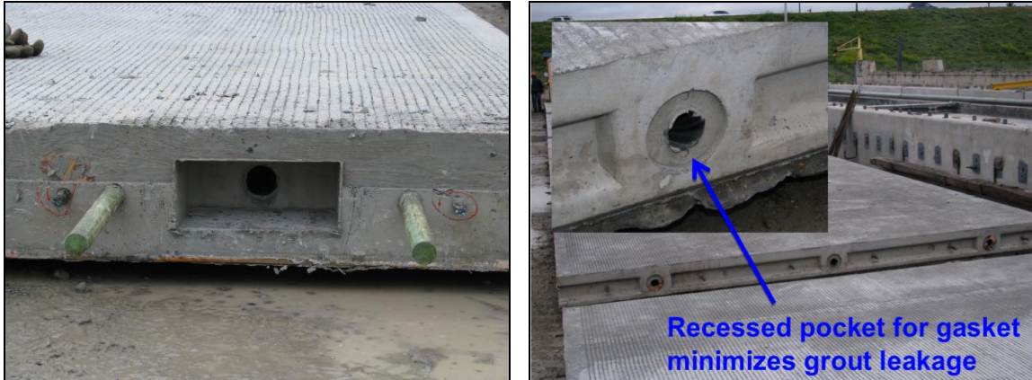
Figure 5 – (a) Blockouts and dowels on end panels only; (b) Keyway and 2-inch diameter PT ducts between PPCP panels
