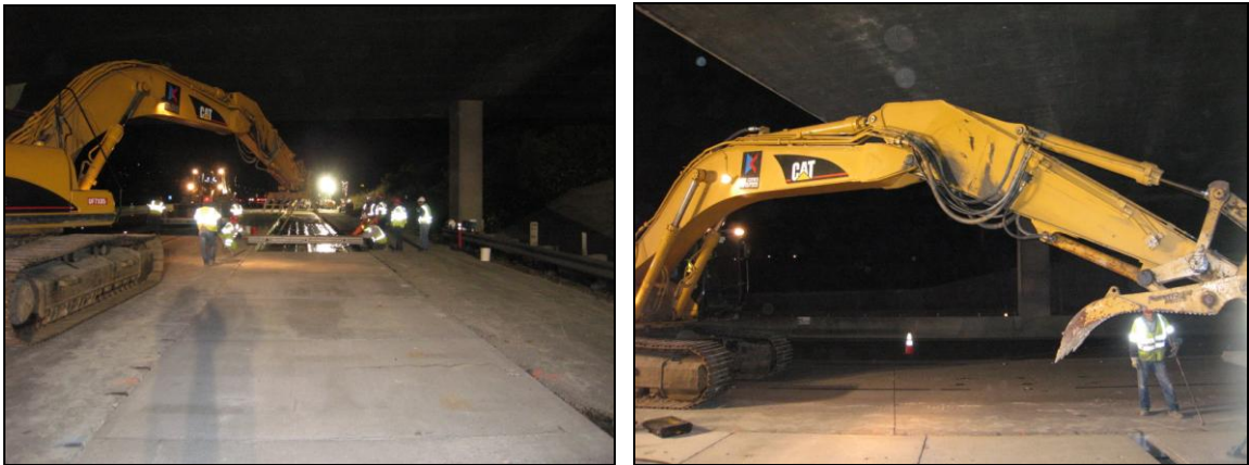
Figure 18 - PPCP installation under a structure (17' clearance)
