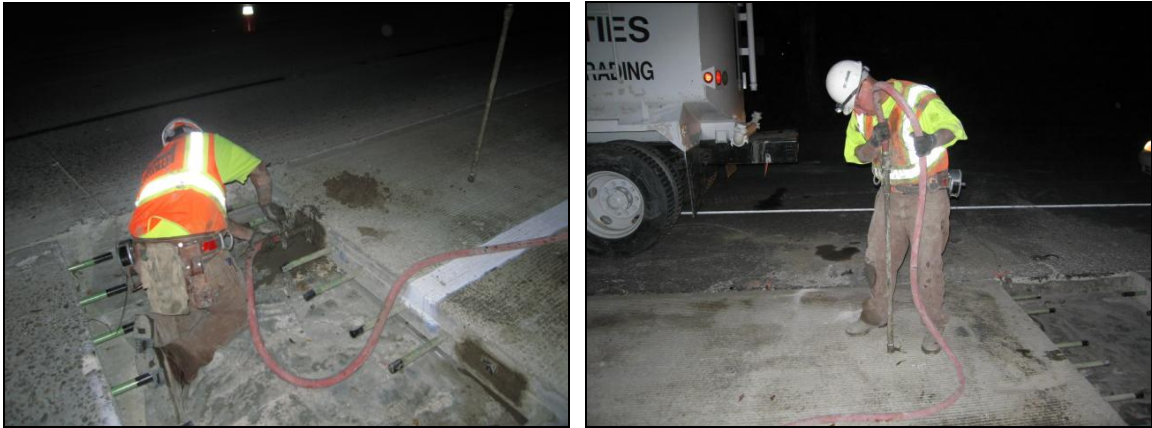
Figure 13 – PT duct and underslab grouting
