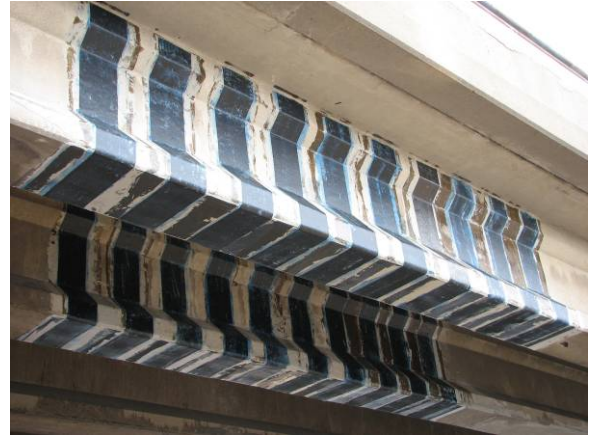
Fig. 15: CFRP Strengthening
