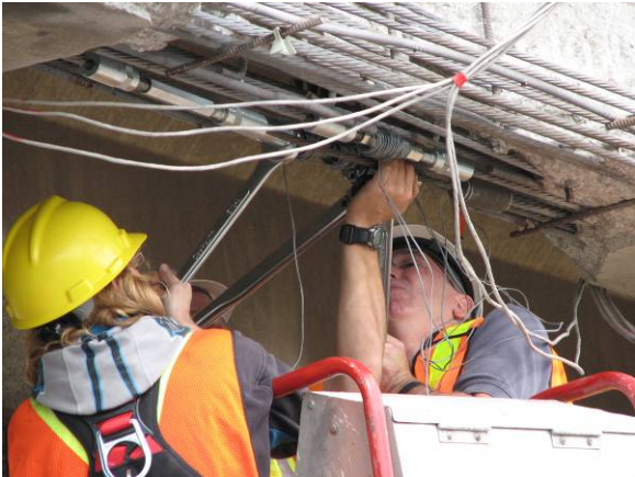
Fig. 21: Tensioning Mechanical Couplers
