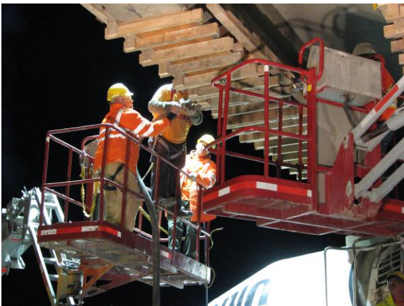
Fig. 12: Pumping SCC
