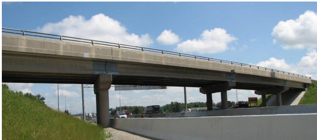
Fig. 1: Highway 401/Dingman Drive Underpass, West Elevation
