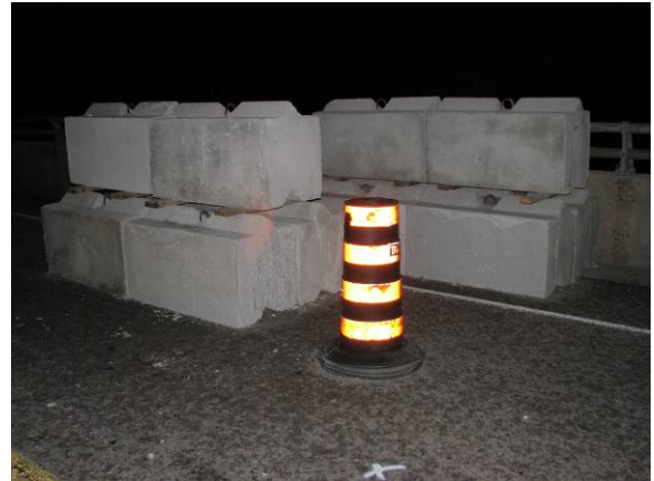
Fig. 22: Preload on Bridge Deck
