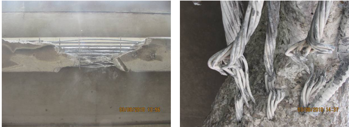
(a) Soffit View
