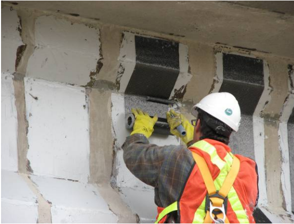
Fig. 14: Installation of CFRP
