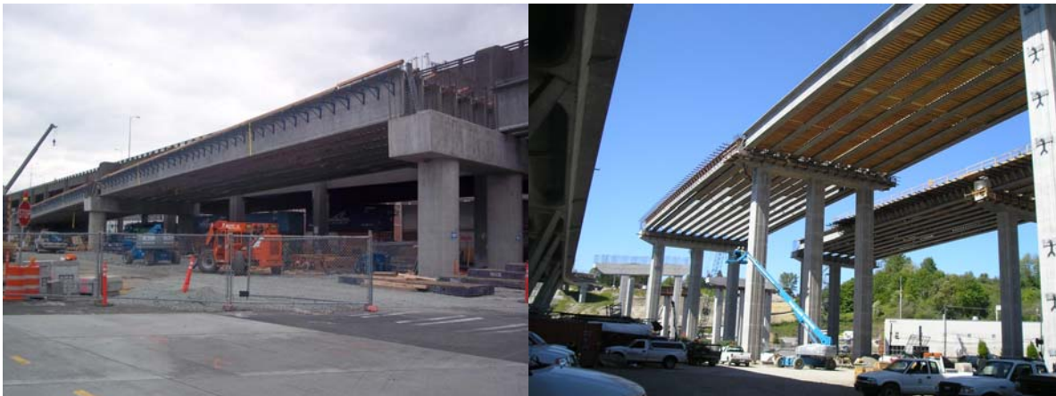
Fig. 9: Erection of WF100G and WF83G Precast Girders
