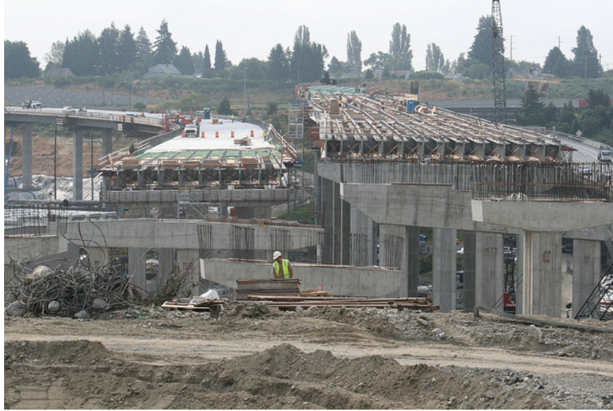
Fig. 1: A Long Span Precast Girder Bridge Project in Washington State
