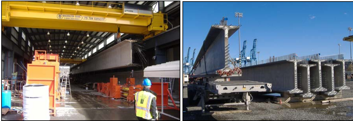
Fig. 7: Long Span Prestressed Girders at the Fabrication Plant and Storage Yard.
