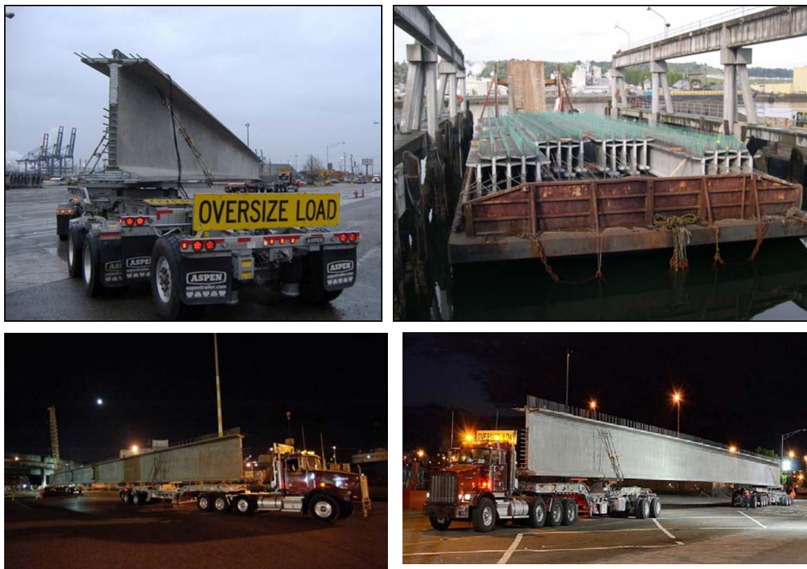
Fig. 8: Shipping of Precast Girders
