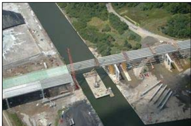
Fig. 4: Erection of Segmental Bulb-Tees Pg#6
