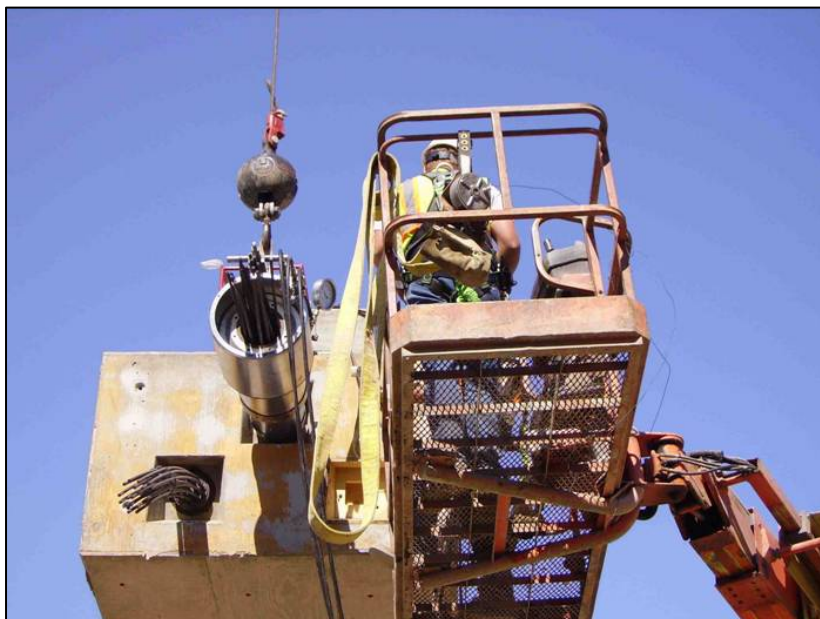
Fig. 10: Post-tensioning of Pier Caps
