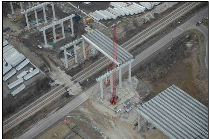
Fig. 3: Erection of 170 ft Prestressed Beams
