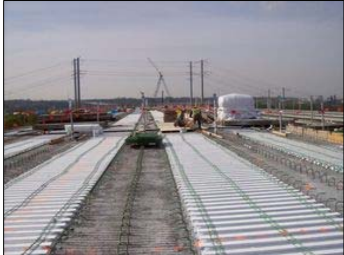
Fig. 8: SIP Forms with Styrofoam
