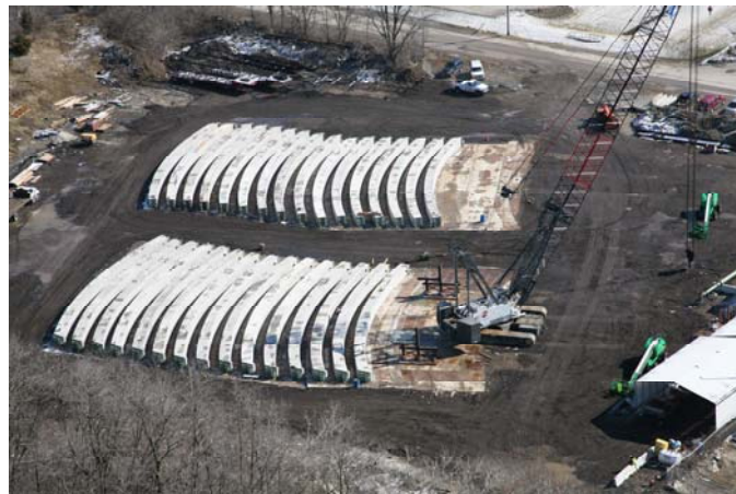
Fig. 17 Finished Arch Segments 18
