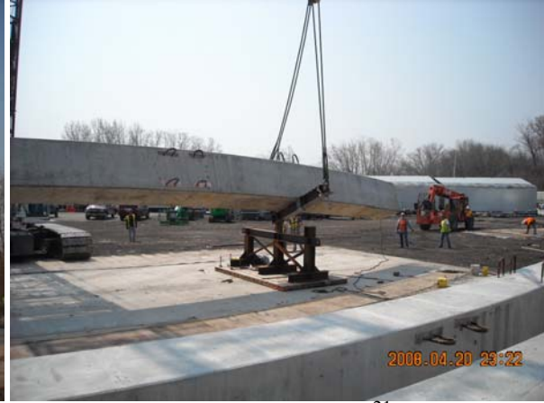
Fig. 20 Arch Segment Rotating 21
