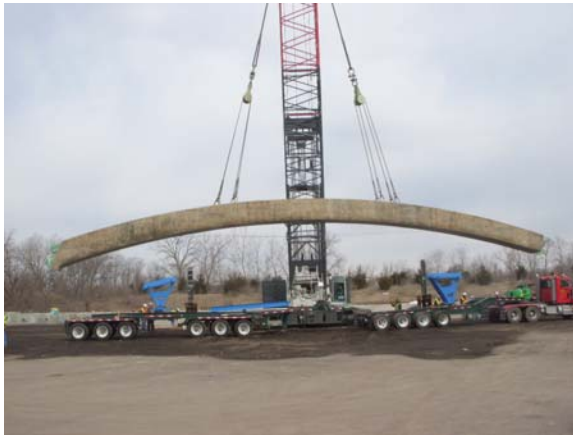
Fig. 21 Arch Segment Lifted onto Truck 23
