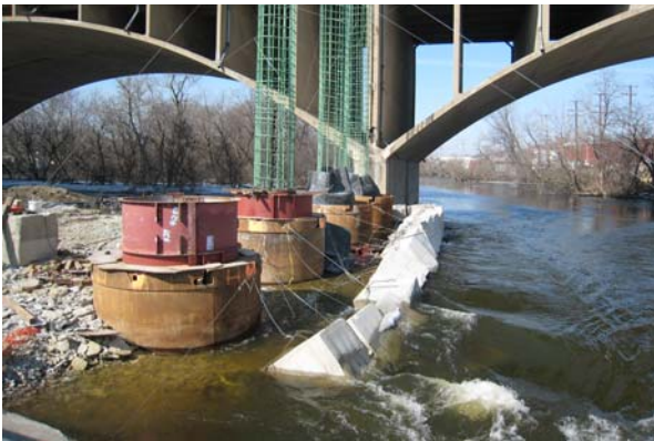
Fig. 3 Pipe Cofferdam for Substructure 4
