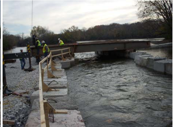
Fig. 6 Temporary Work Bridge 7
