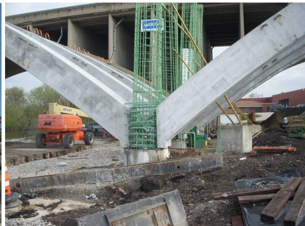
Fig. 12 Fox River Bridge Arch Base 13
