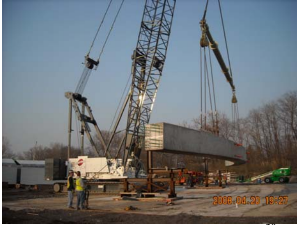
Fig. 19 Crane Lifting Segment to Device 20
