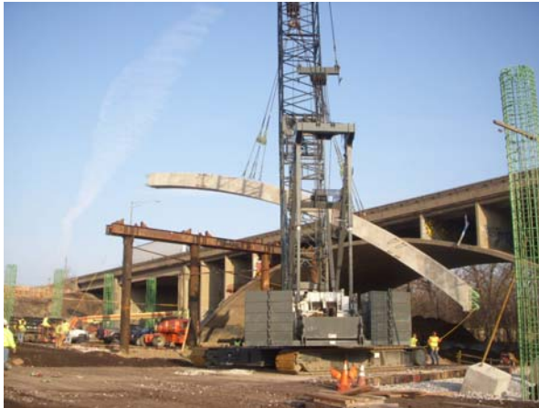
Fig. 23 Lifting Arch Segment 25
