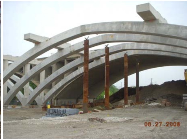
Fig. 29 Completed Spandrels 31
