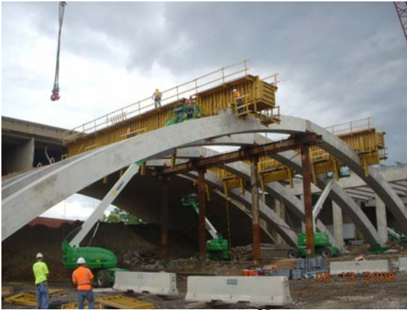
Fig. 28 Forming of Spandrel 30
