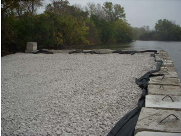
Fig. 5 Temporary Work Platform 6
