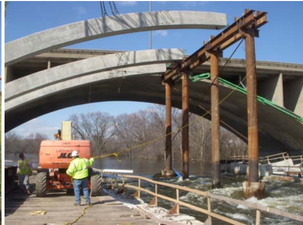
Fig. 24 Positioning Arch Segment 26
