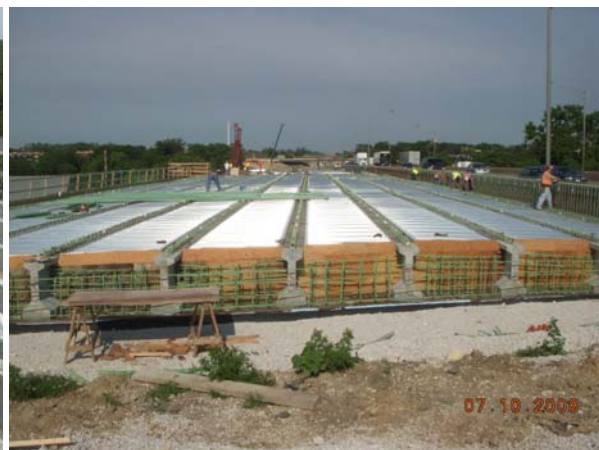
Fig. 10 Precast Beams & SIP Metal Forms 11
