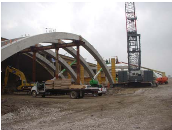
Fig. 25 Continuous Arch Span 27
