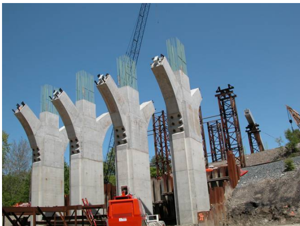
Fig. 11 Cleveland Zoo Bridge Arch Base 12
