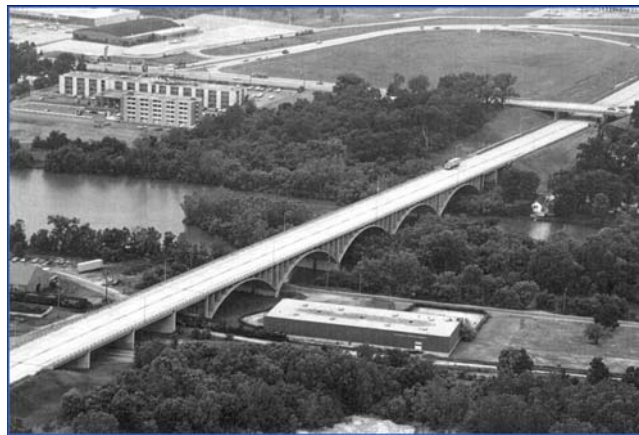
Fig. 1 Original Bridge over the Fox River 1
