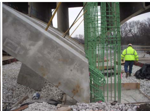
Fig. 26 Arch Thrust Block Rebar 28
