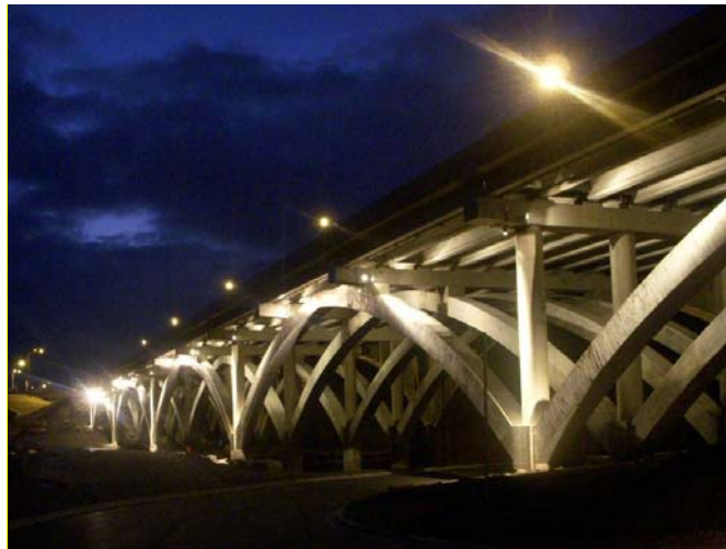
Fig. 30 Completed I-88 Bridge over the Fox River 32
