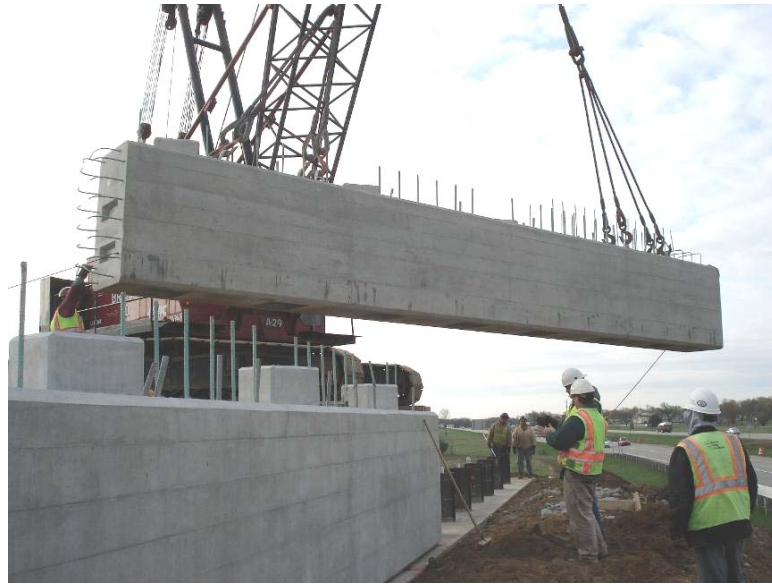
Fig. 10 Erection of Precast Integral Abutment Pile Cap 25
