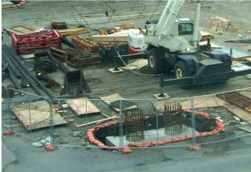
Figure 4 Shaft Reinforcement in the Hinge Zone
