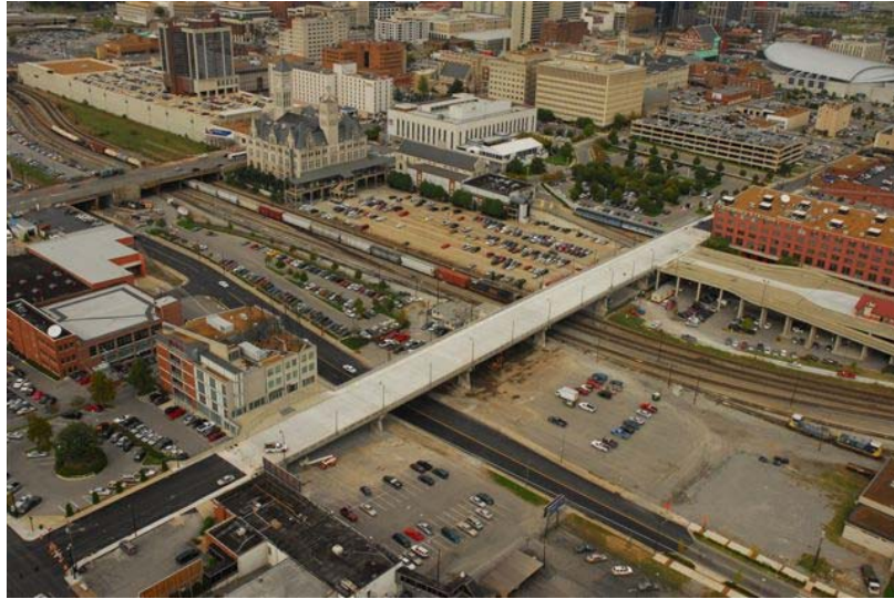
Figure 2 7-span Jointless Viaduct Replacement
