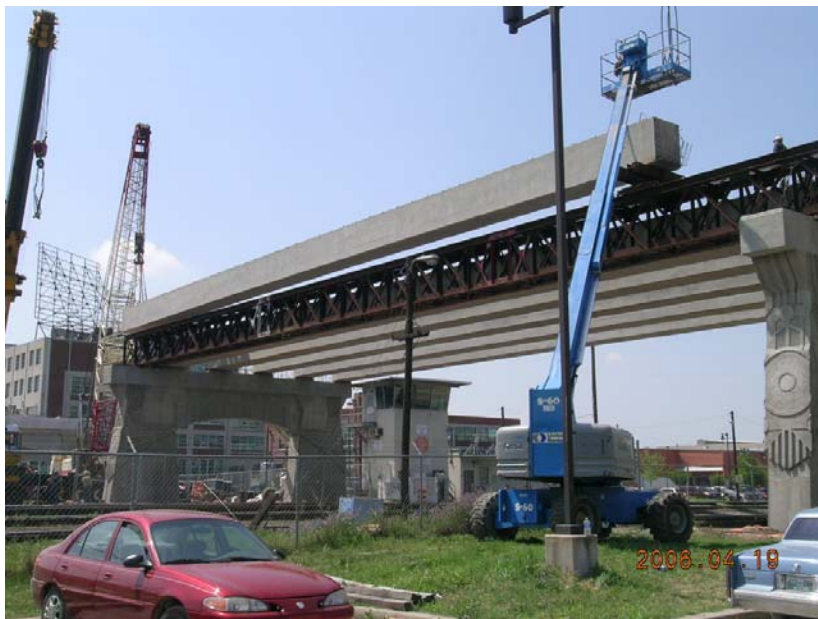
Figure 7 Launching of Beams
