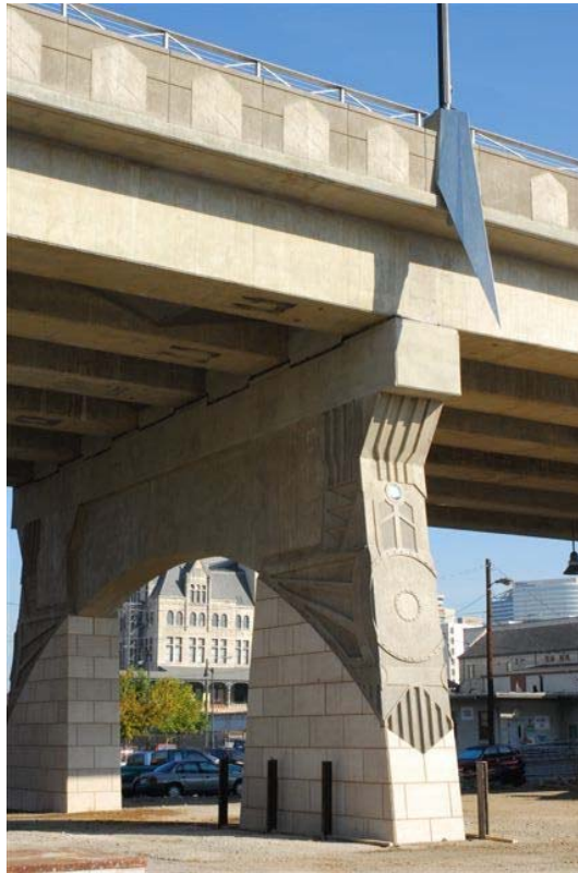
Figure 5 Architectural Bents and Sconces
