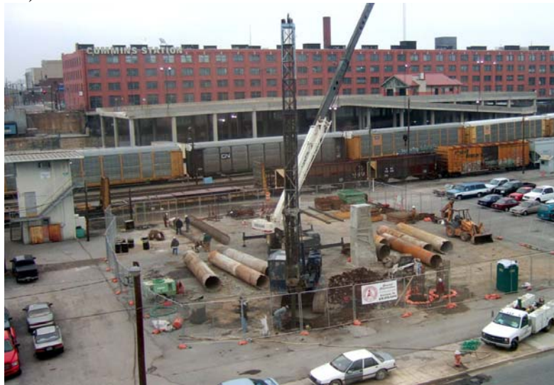
Figure 3 42-in. Diameter Drilled Shafts
