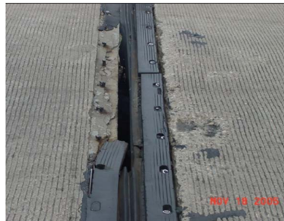
Broken Joint
