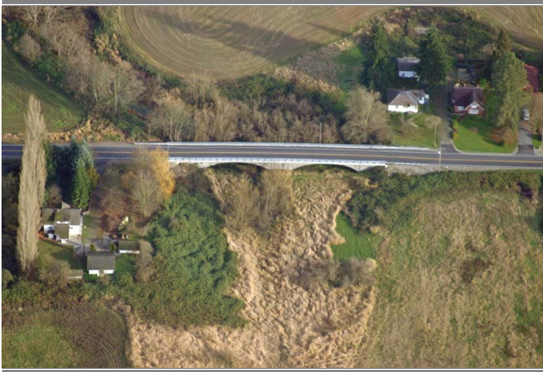
Figure 9. Aerial View of the New Bridge
