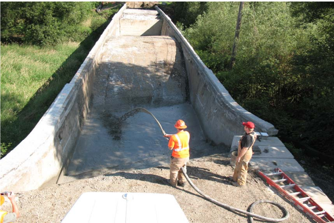
Figure 5. Backfill with Low Density Cellular Concrete
