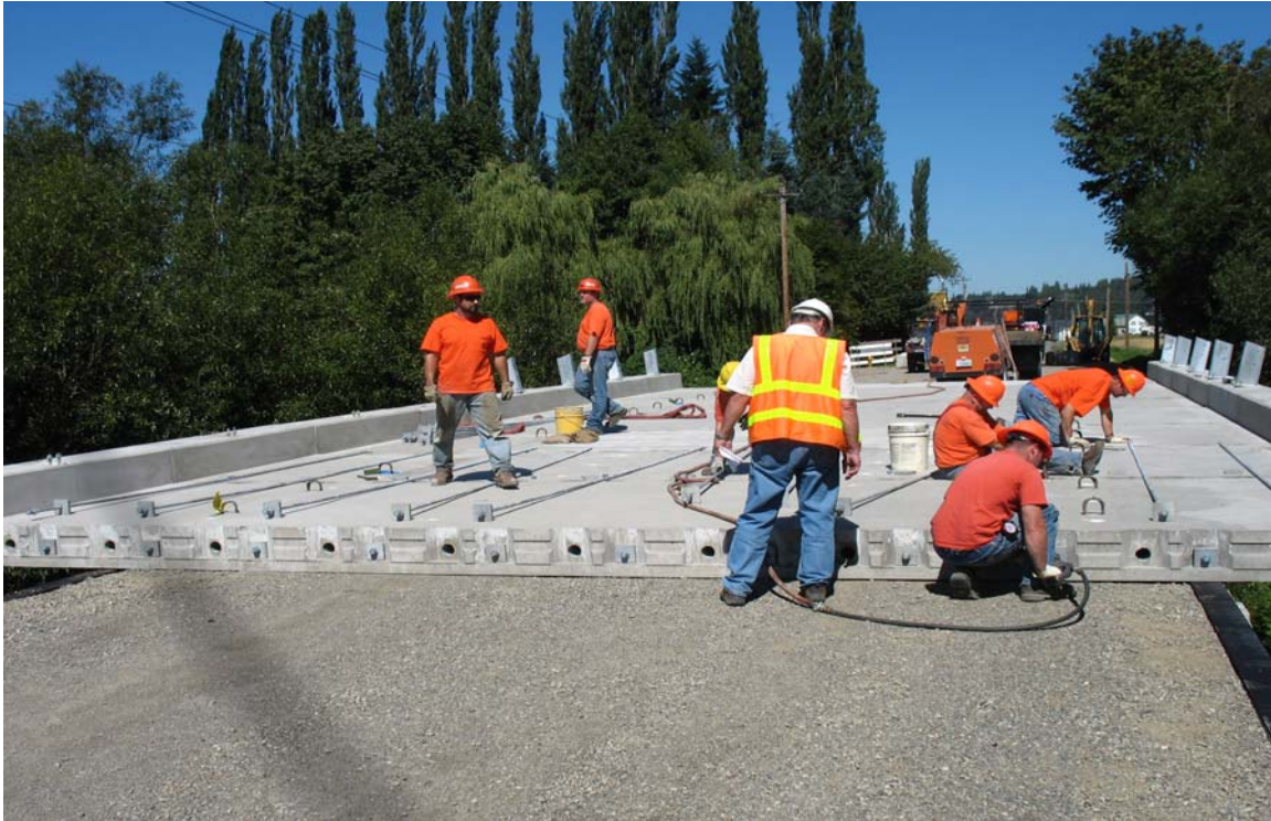
Figure 6. Lay the Precast Concrete Deck Planks
