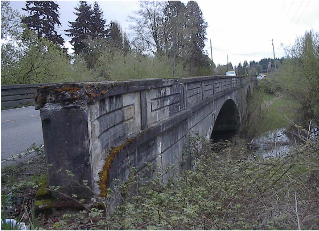
Figure 3. Existing Bridge (Looking South)
