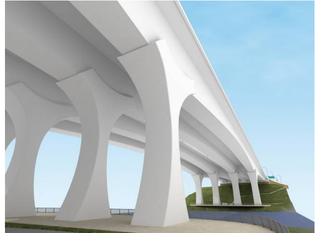
Figure 15 – Each box girder is supported on its own column and own set of drilled shafts
