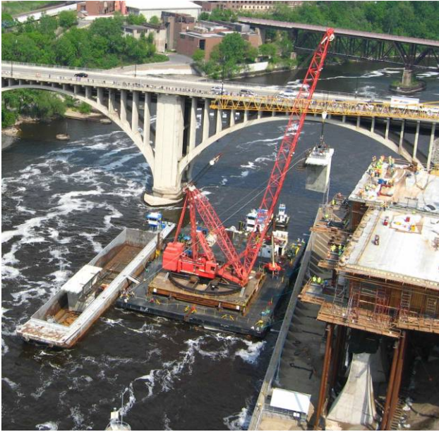
Figure 13 – First Precast Erection May 25, 2008
