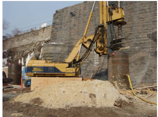
Figure 6 – Drilling Shafts from Land
