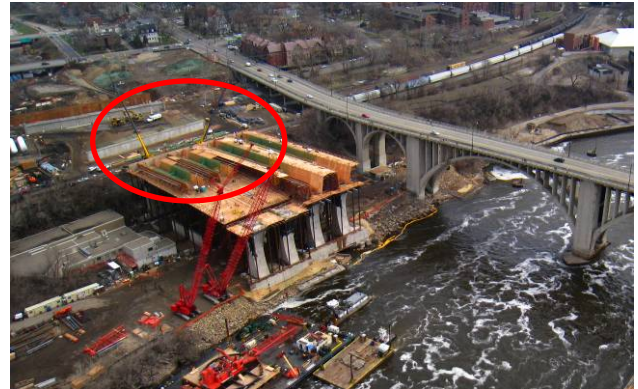
Figure 12 – Railway on Bluff at North Side of Bridge
