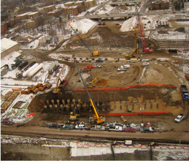
Figure 3 – Footings on North side of River
