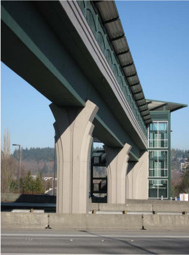
Figure 8. Column details are visually dominant over the superstructure.
