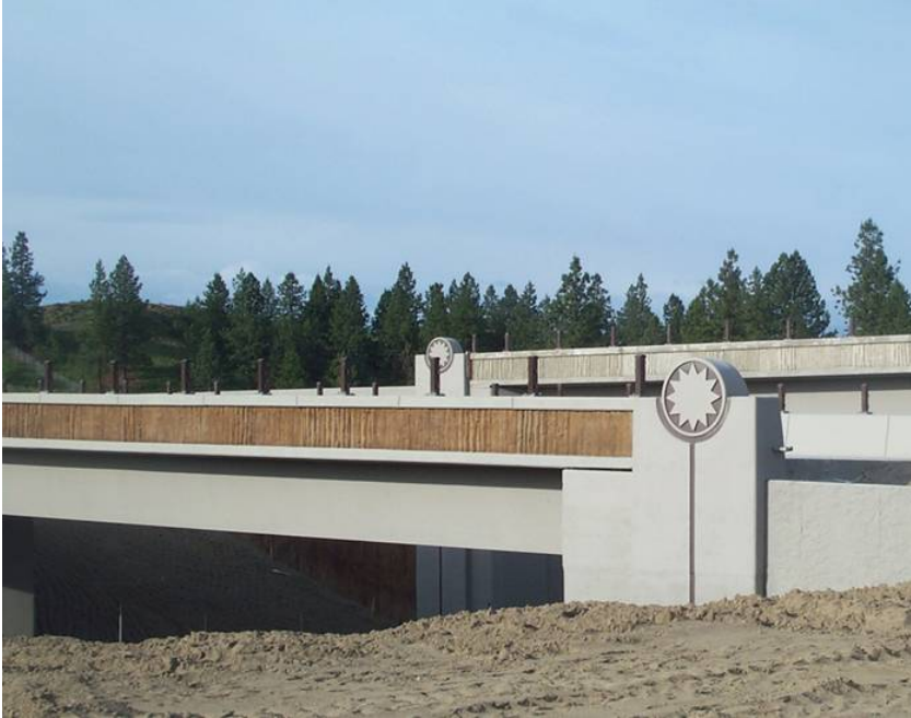
Figure 7. Abutment details overshadow the superstructure type.
