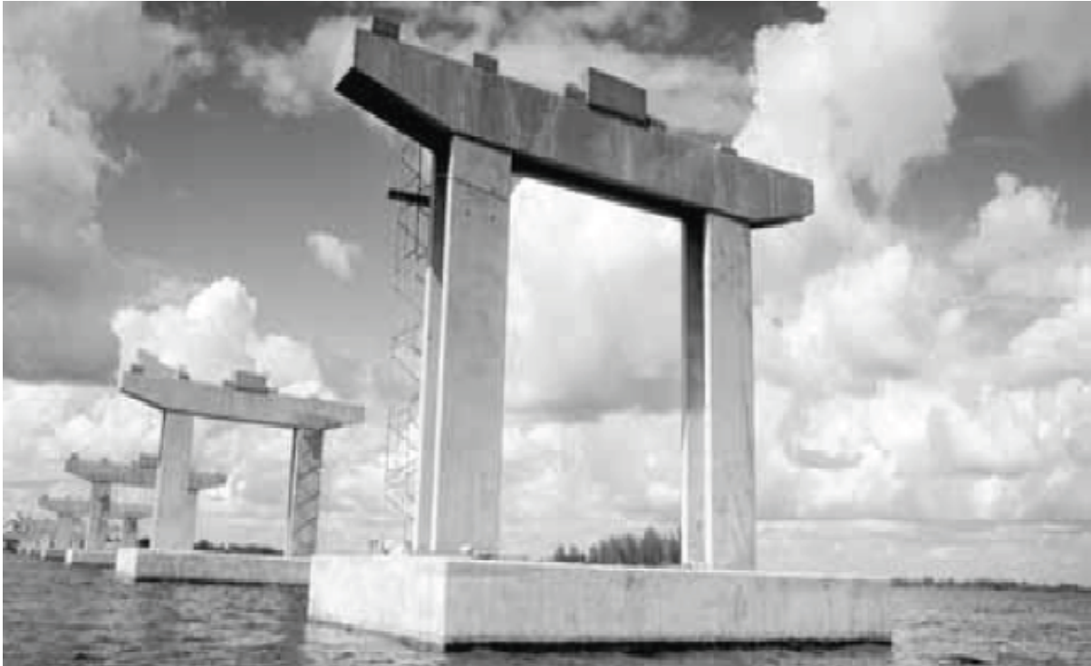
Fig. 1 Edison Bridge Ft. Meyers, Fla, Showing Precast Concrete Columns and Caps
