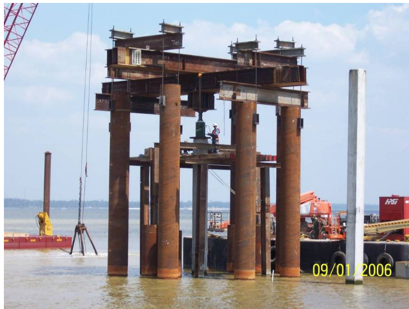
Fig. 4 Axial Static Load Test of 24 inch Pile
