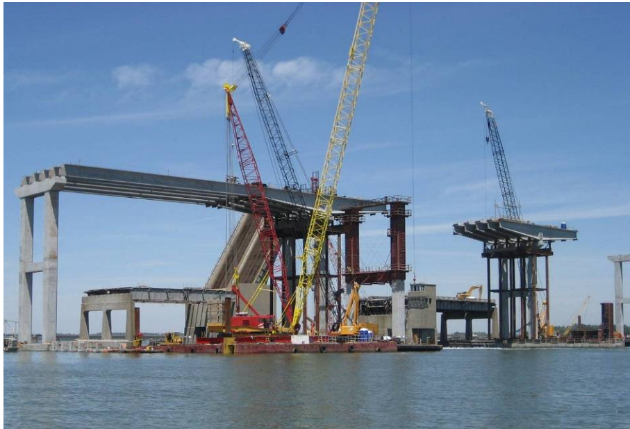
Fig. 10 Erection of the Navigation Unit
