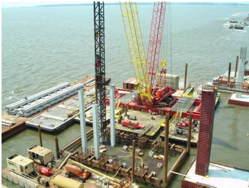
Fig. 6 Pile Installation
