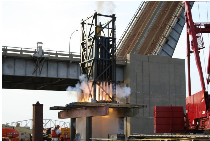
Fig. 5 Statnamic Axial Load Test of 30 inch Pile
