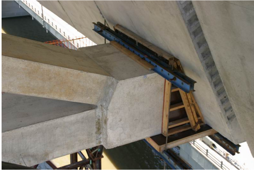
Fig. 8 Forming for the delta frame bottom corner closure pours.
