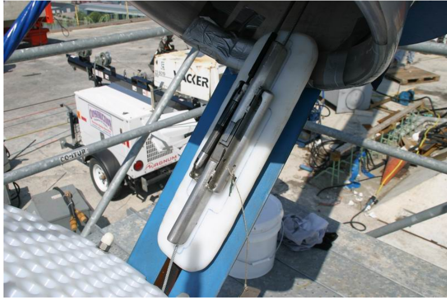
Fig. 18 Shuttle used during stay strand installation.
