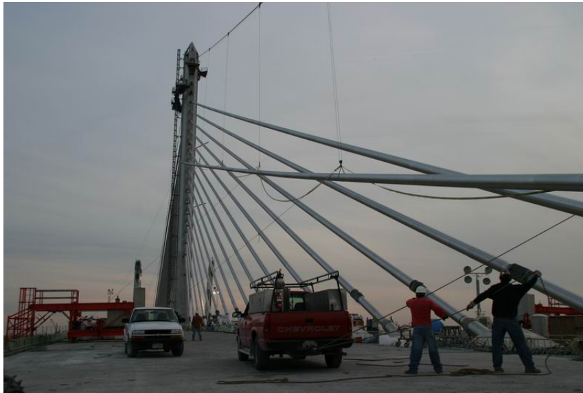
Fig. 16 The highline system lifts the sheathing into place for Stay 18.
