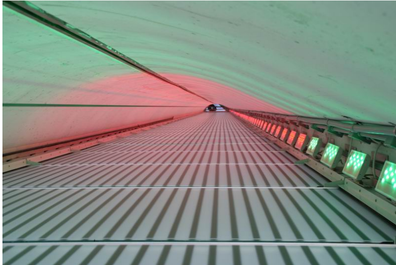
Fig. 22 LED light fixtures reflect red and green light off of the curved pylon concrete.
