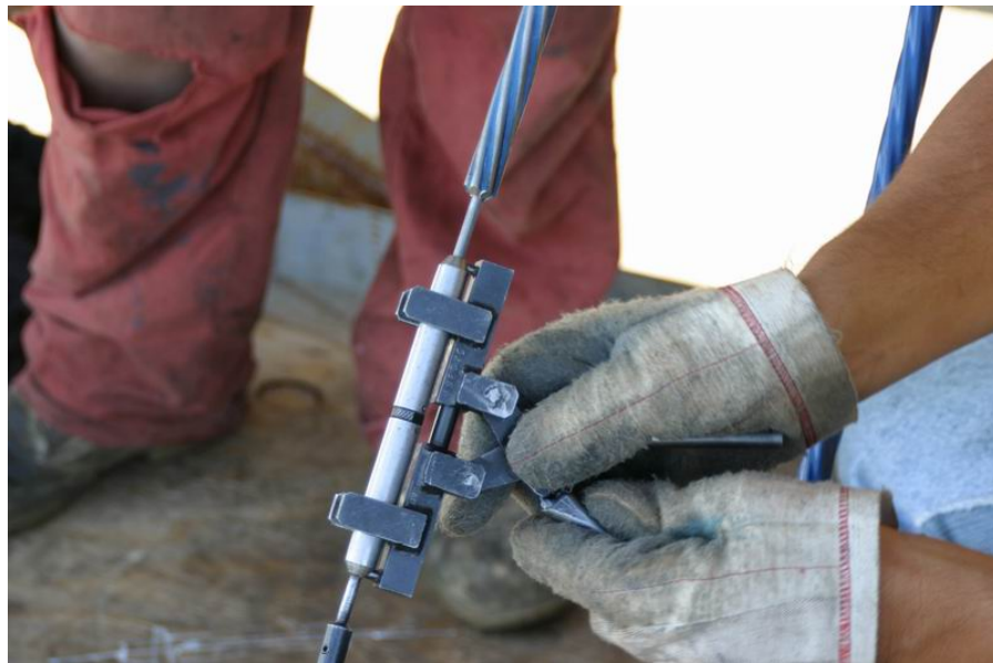
Fig. 17 Kingwire coupler and disconnection tool.
