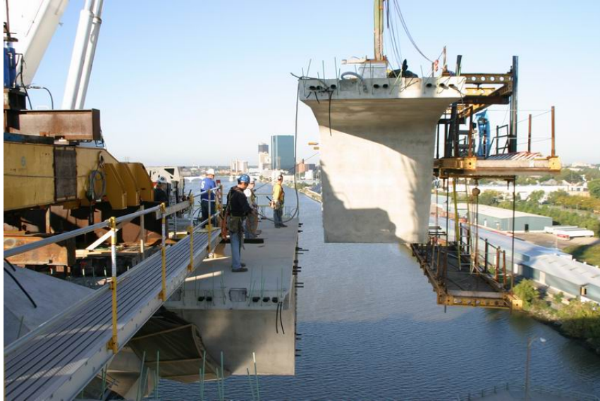
Fig. 6 Erection of precast superstructure segments in cantilever.
