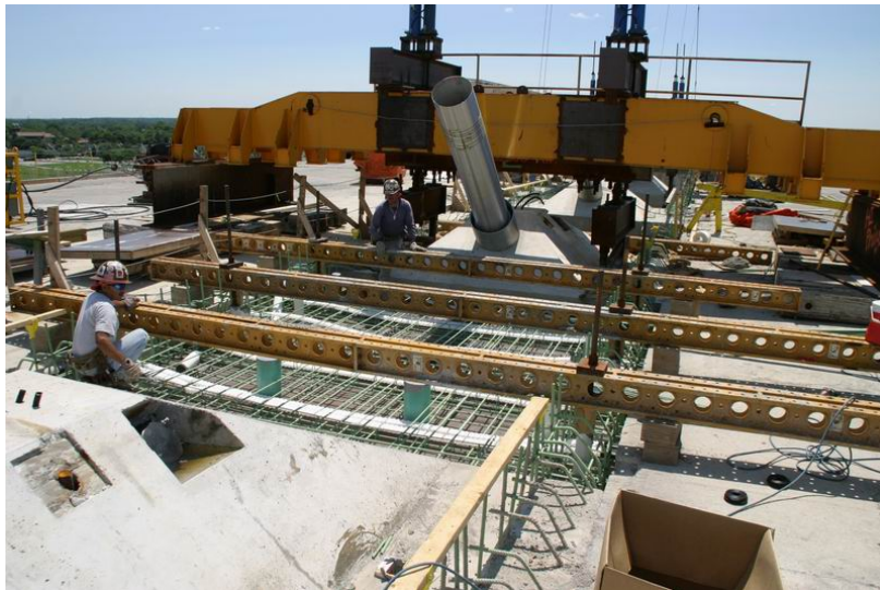
Fig. 9 Formwork, reinforcement, and transverse post-tensioning for the median slab.
