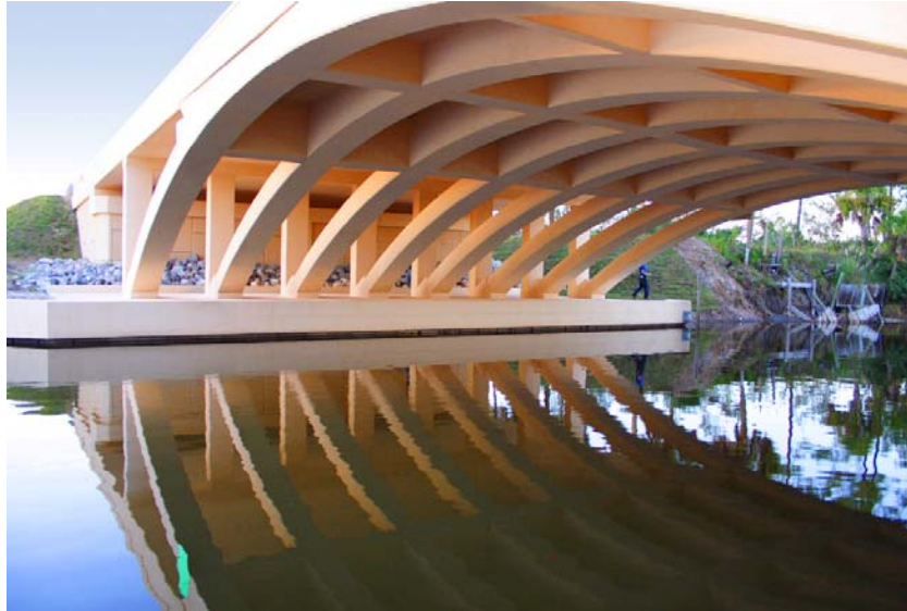
Figure 10 – Arch Diaphragms
