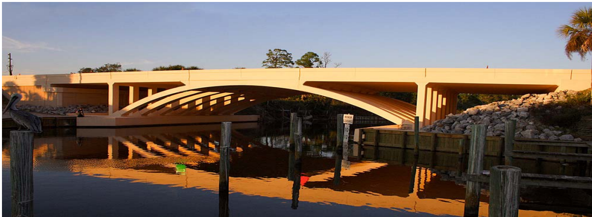
Figure 14 – Completed Arch Elevation
