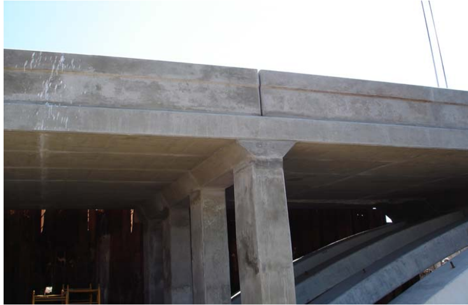
Figure 13 – Flat Slab at Transverse Beam
