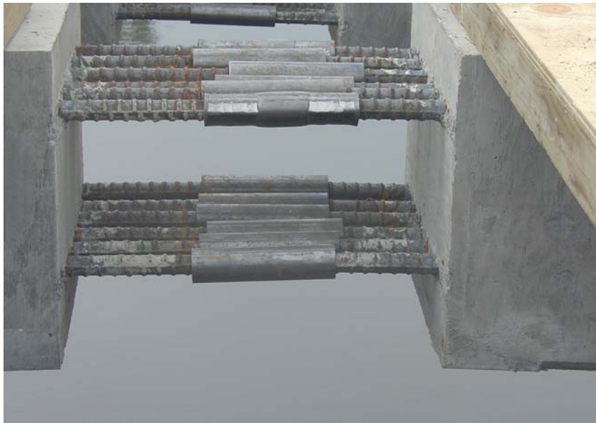
Figure 9 – Mechanical Splice at Arch Crown
