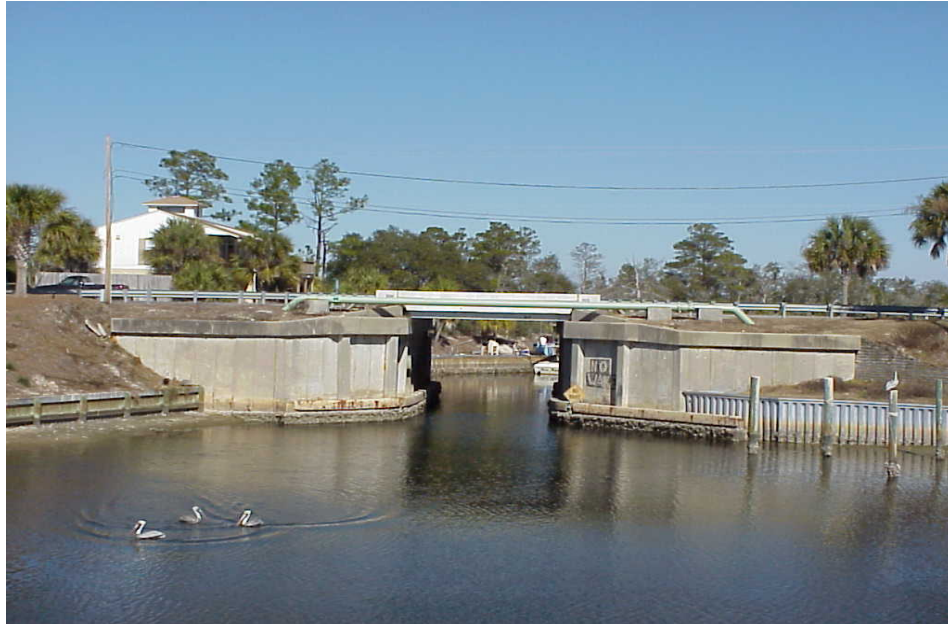
Figure 2 – Existing Site Conditions
