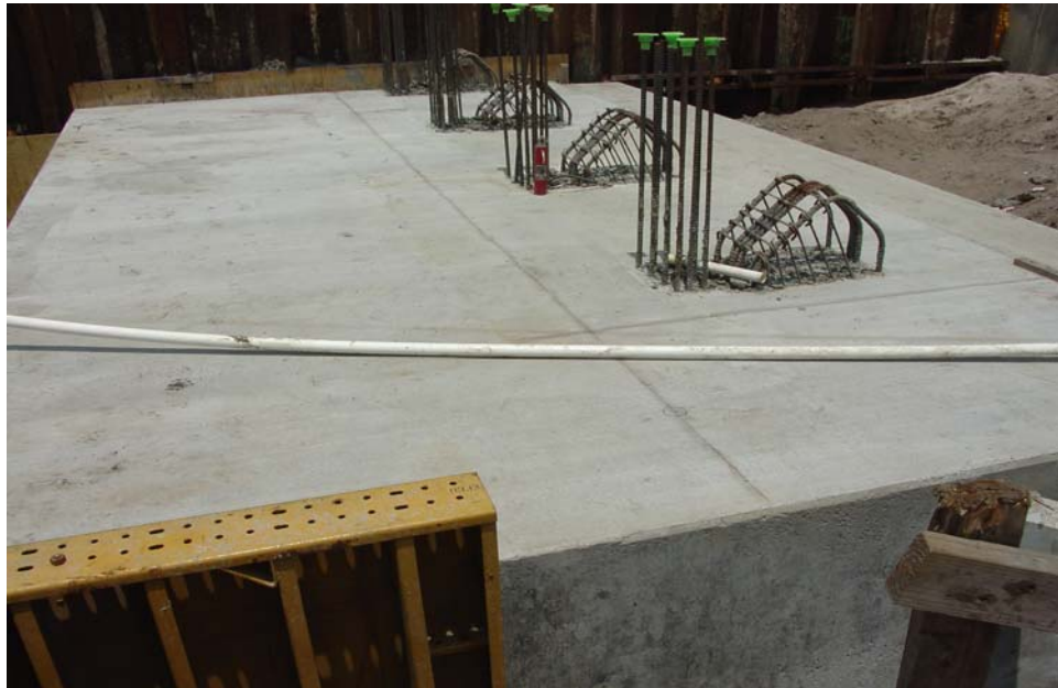
Figure 12 –Foundation after Form Removal
