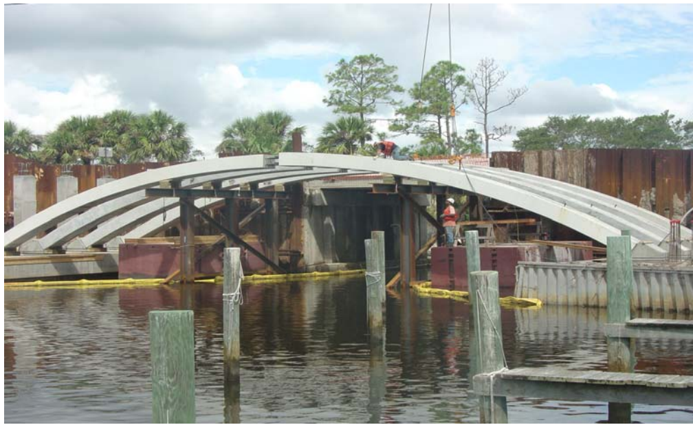
Figure 5 – Arches on Temporary Supports –Phase I
