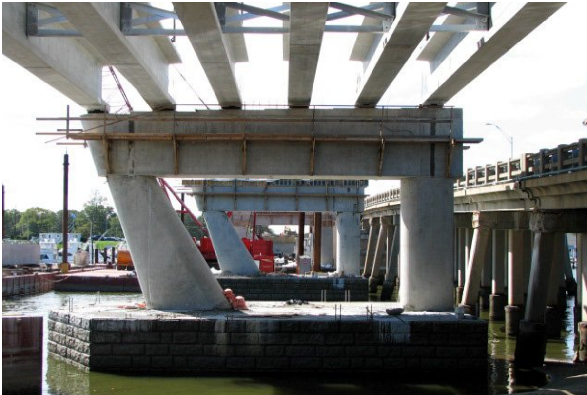
Fig. 14. Span 6 PCEF Bulb Tee girders have been erected.
