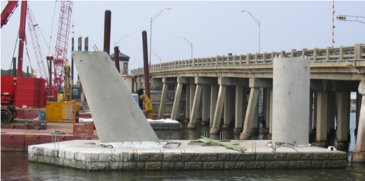
Fig. 12. The first precast pier columns have been erected.
