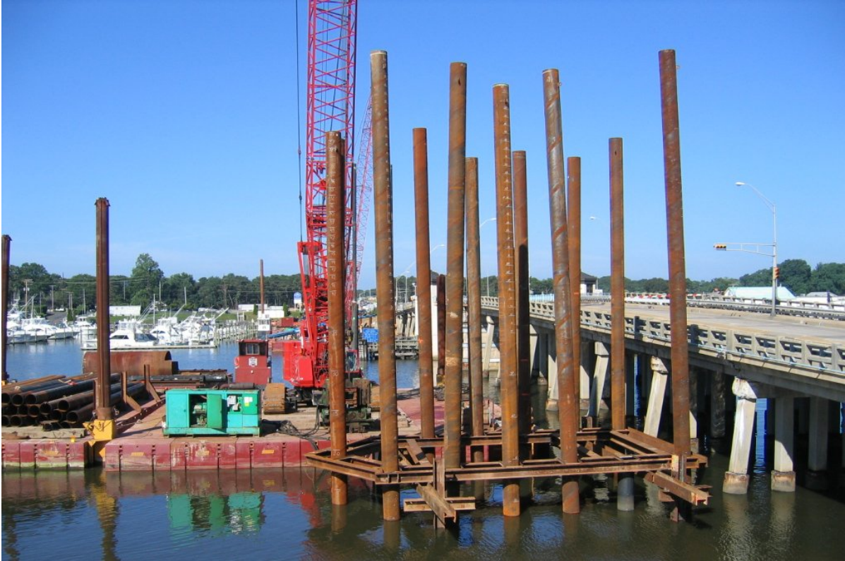
Fig. 7. Perimeter piles driven with a template.
