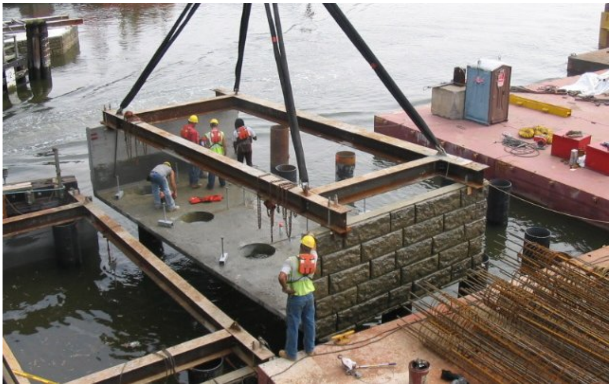
Fig. 9. Precast cofferdam section being hoisted into place.
