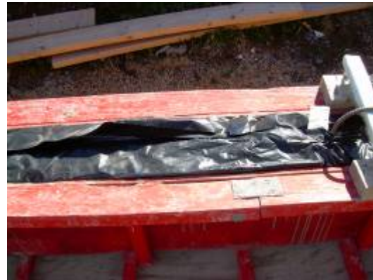
Fig. 5 Beam Sealed after Casting
