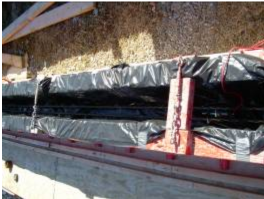
Fig. 4 Formwork before Casting
