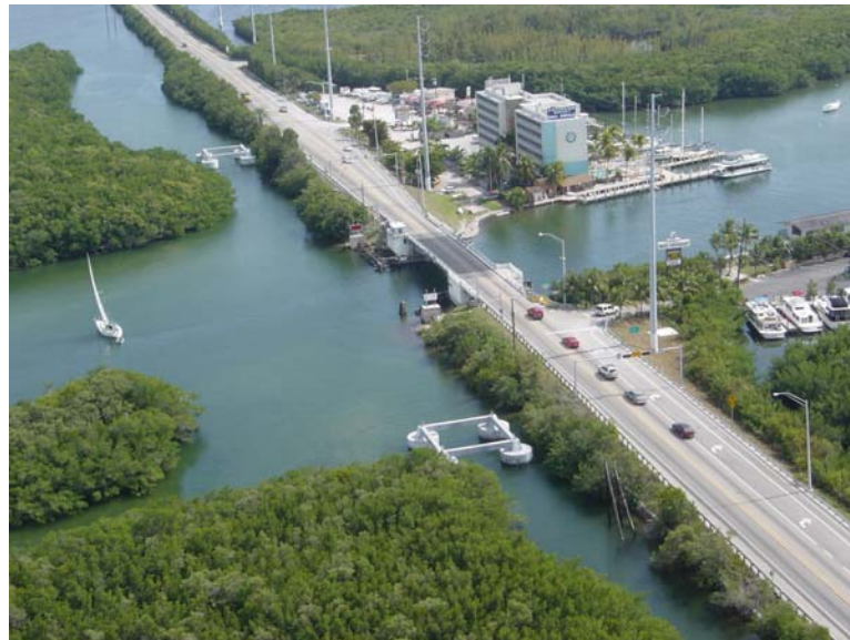
Figure 2 – Existing Bridge and Causeway
