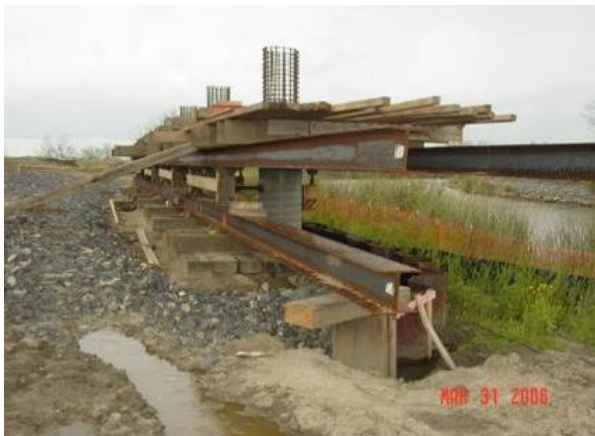
a) Temporary Falsework
