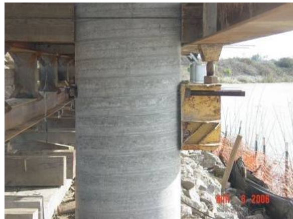
b) Falsework Attachment Detail
