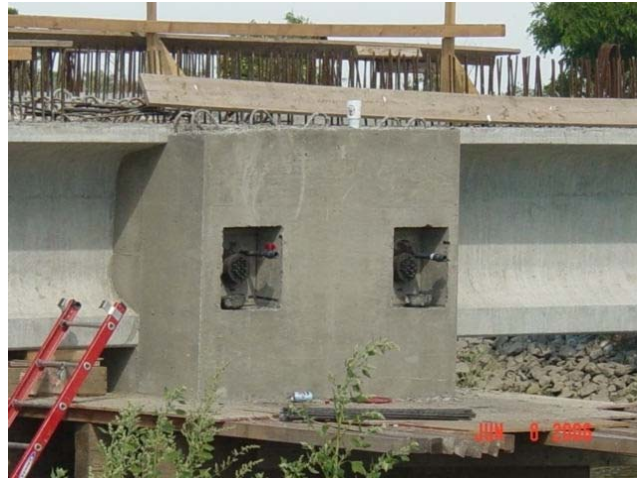
Fig. 3 Transversely Post-tensioned Integral Bent Cap
