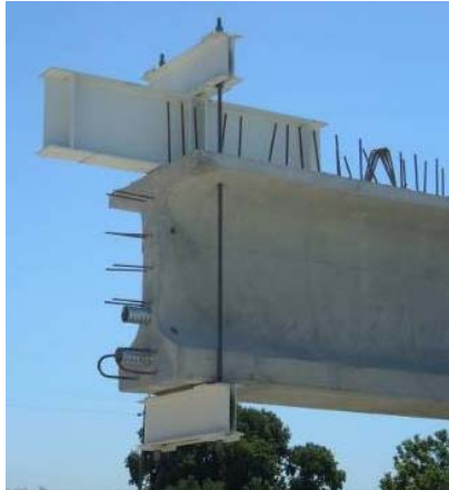
Fig. 5 Strongback Used to Support the Middle Span Drop-in Segment
