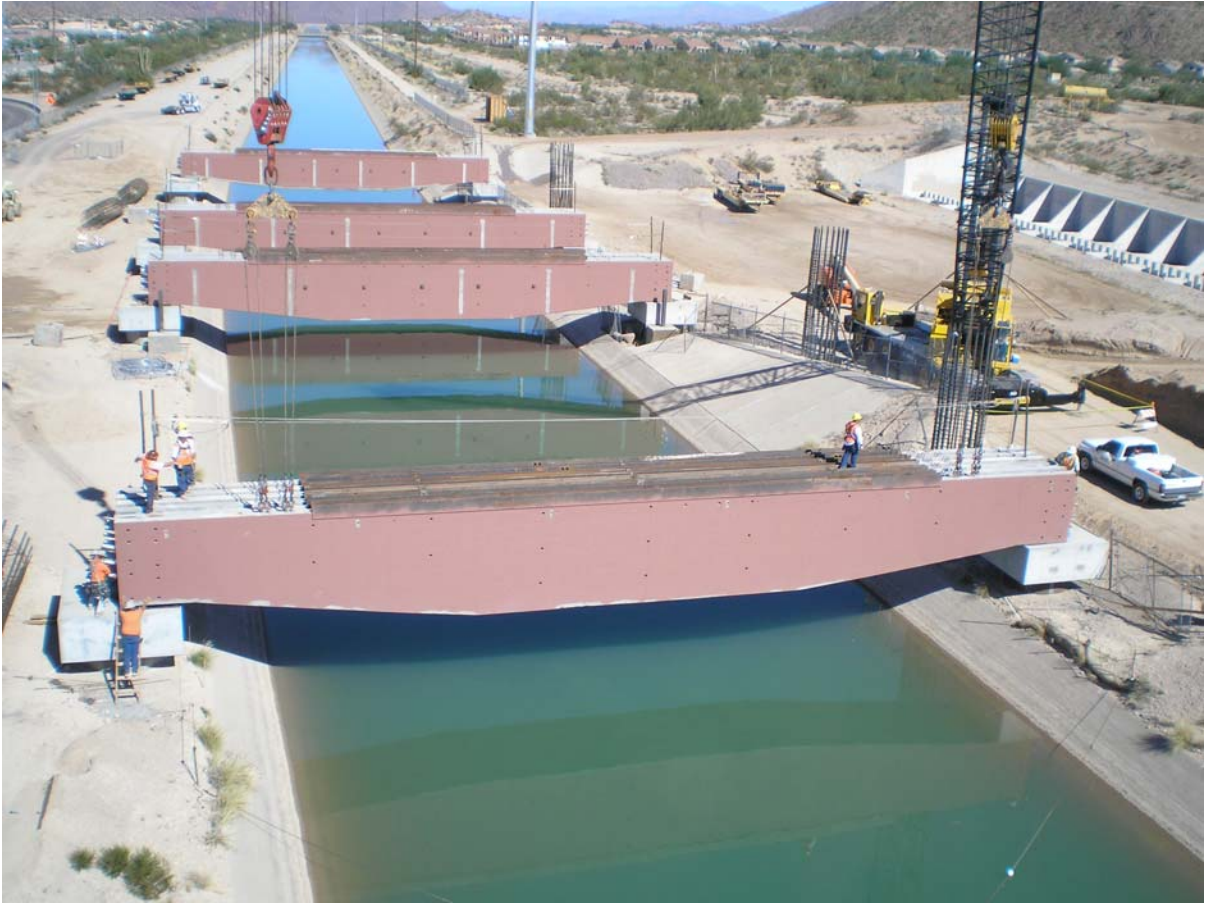
Fig. 7 – Special straddle assemblies normal to the CAP Canal.
