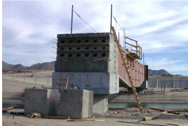
Fig. 11 – End block with 18 post-tensioning ducts.
