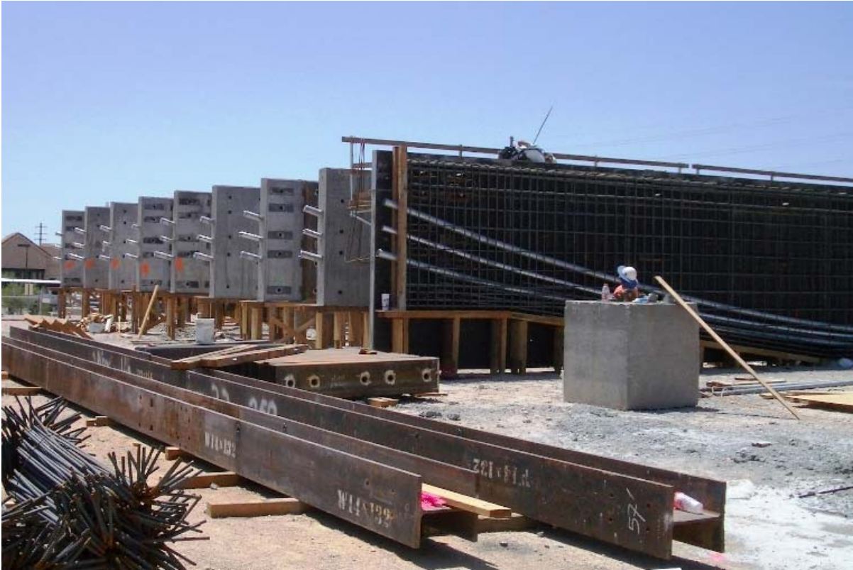
Fig. 13 – Precast plies produced on-site eliminate truck haul.
