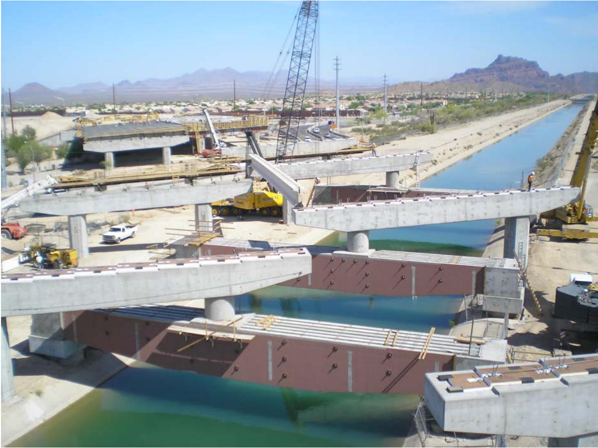
Fig. 2 – Looking Back Station at three of the four special straddling piers.
