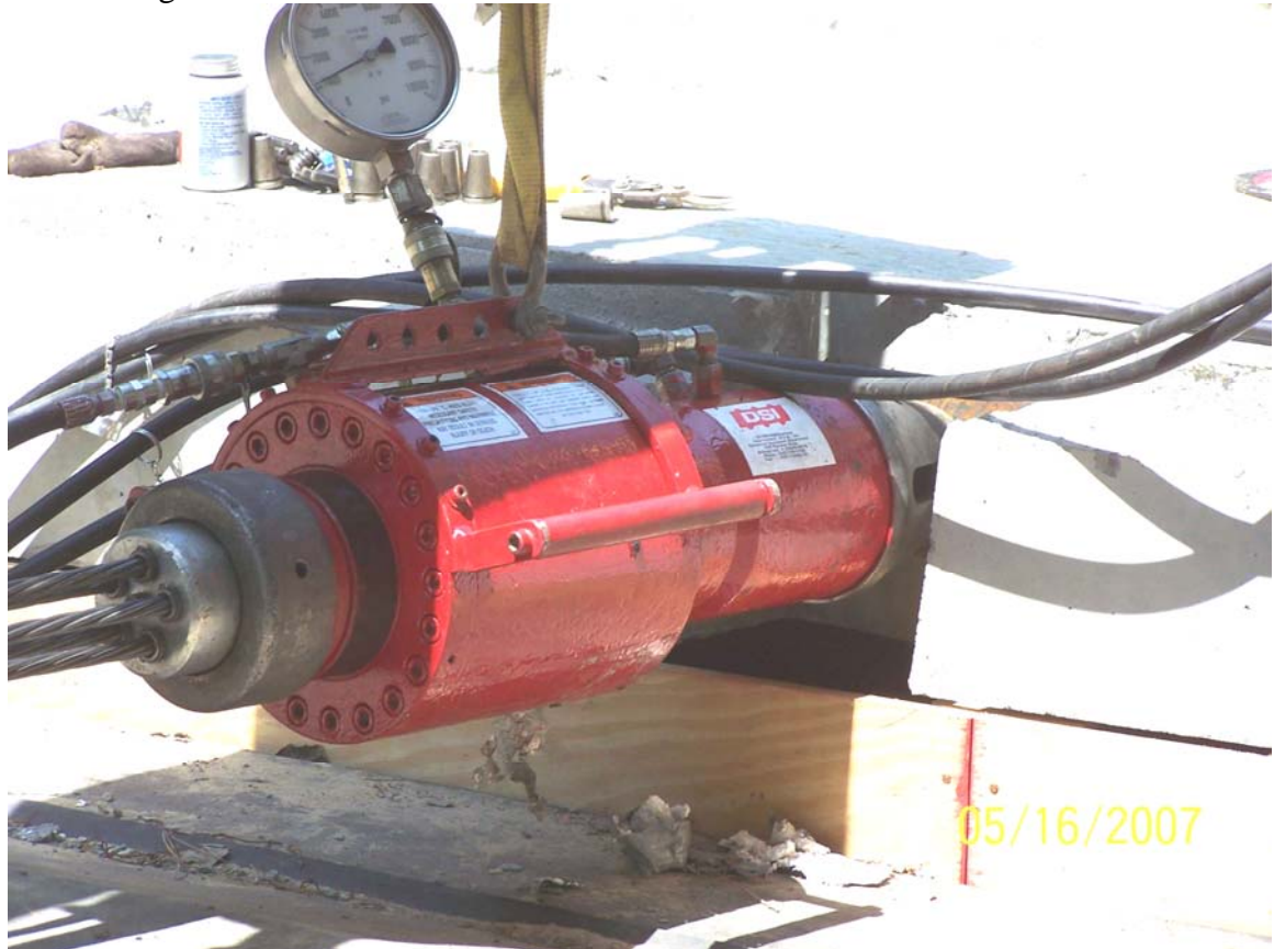
Figure 10 – The Portable jack can easily pull all five 0.6” strands
