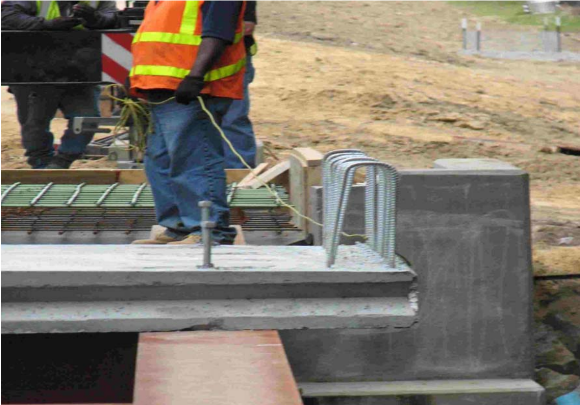
Figure 3 -- Panel resting directly on Leveling bolts and girder top flange
