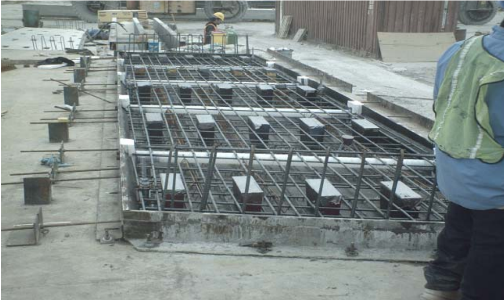
Figure 5 -- Panel and blockout formwork during fabrication
