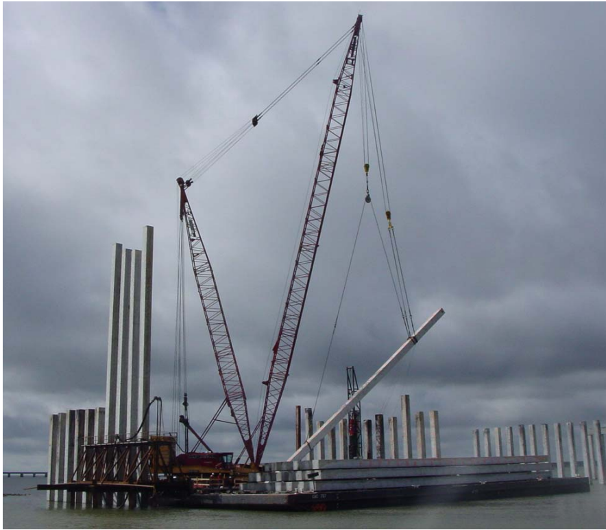
Fig. 3 Two point lofting of 133 ft, 36 in. pile at Bent 57
