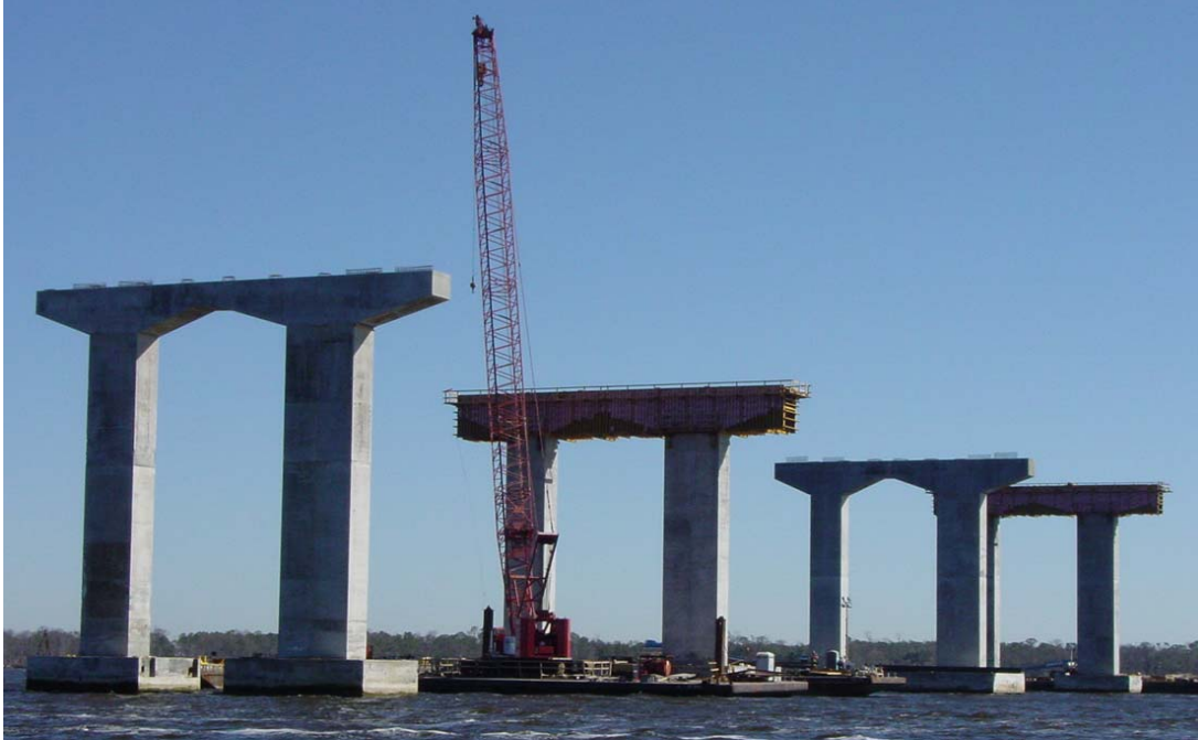
Fig. 5 Completed waterline footings, Bents 37-40
