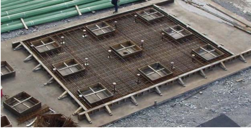
Fig. 8 Fabrication of a typical precast soffit slab.
