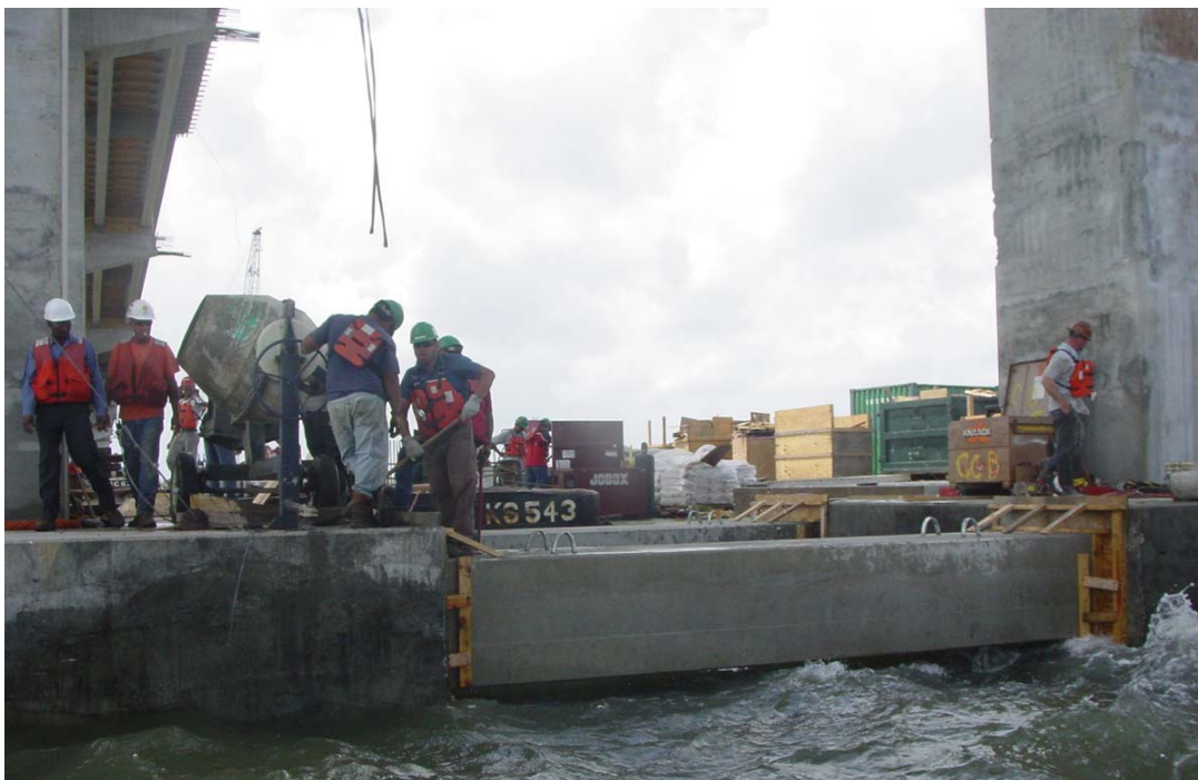
Fig. 10 Precast struts joining the individual footings at Bent 37
