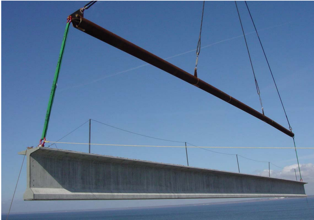
Fig. 11 Rigging configuration of typical 154 ft BT-78
