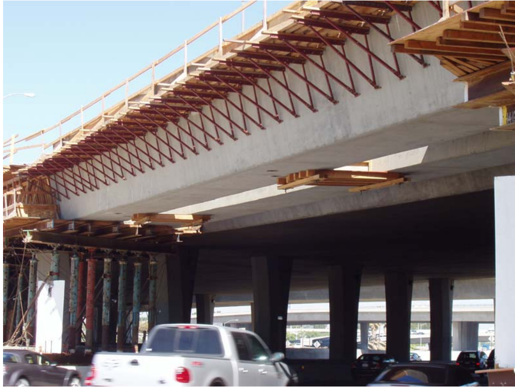
Fig. 8 Deck and intermediate diaphragm forms are suspended from the precast girders.
