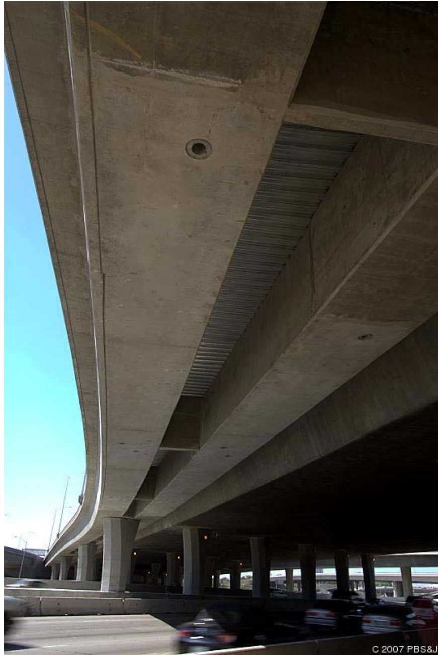
Fig.1 Curved precast concrete bathtub girders span the northbound lanes of I-5.
