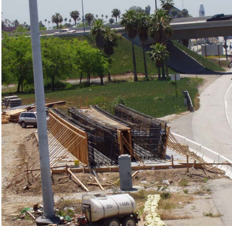
Fig. 6 Precast Bathtub Girder Casting Bed.
