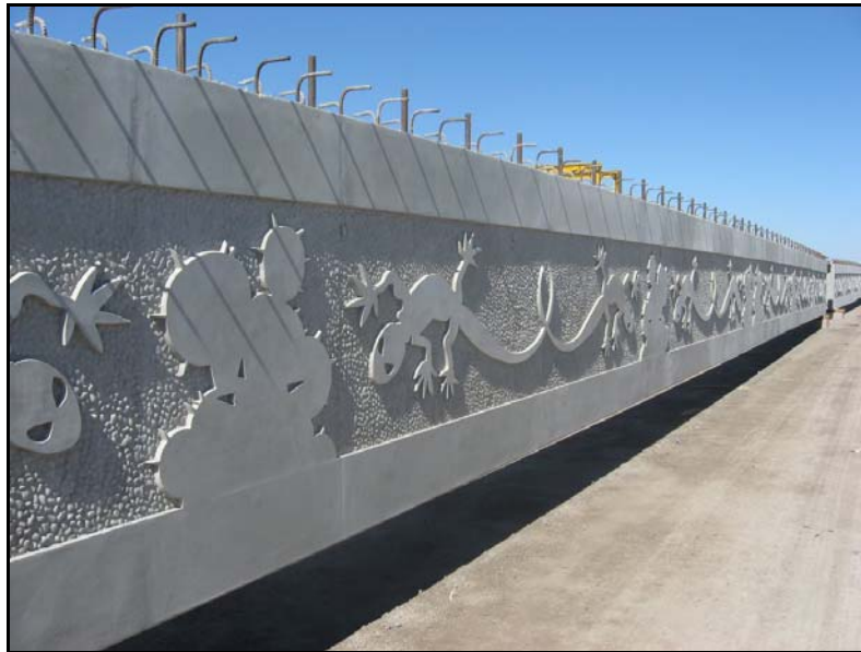
Figure 10: Exterior Girder with Embedded Gecko & Cacti Pattern
