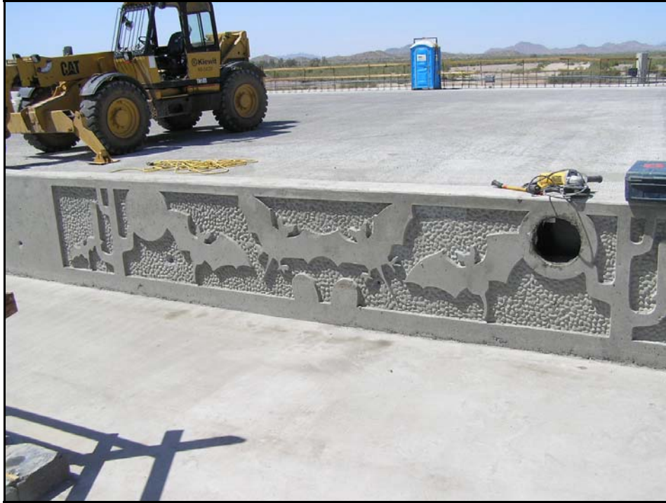
Figure 13: Relief Pattern on Back Face of Barrier
