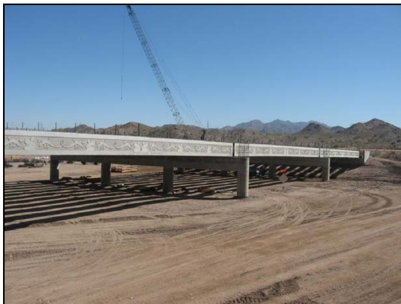
Figure 11: Construction prior to Deck Pour
