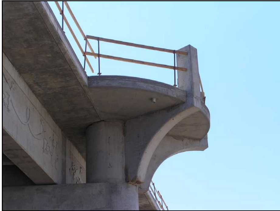
Figure 12: Pedestrian Alcove with Precast Corbels
