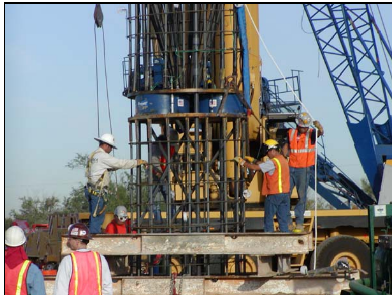
Figure 4: Drilled Shaft Load Test per Osterberg Cell Method
