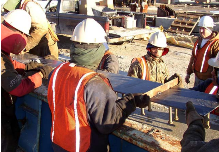
Figure 2 Placement of the Plates in Girder 2.
