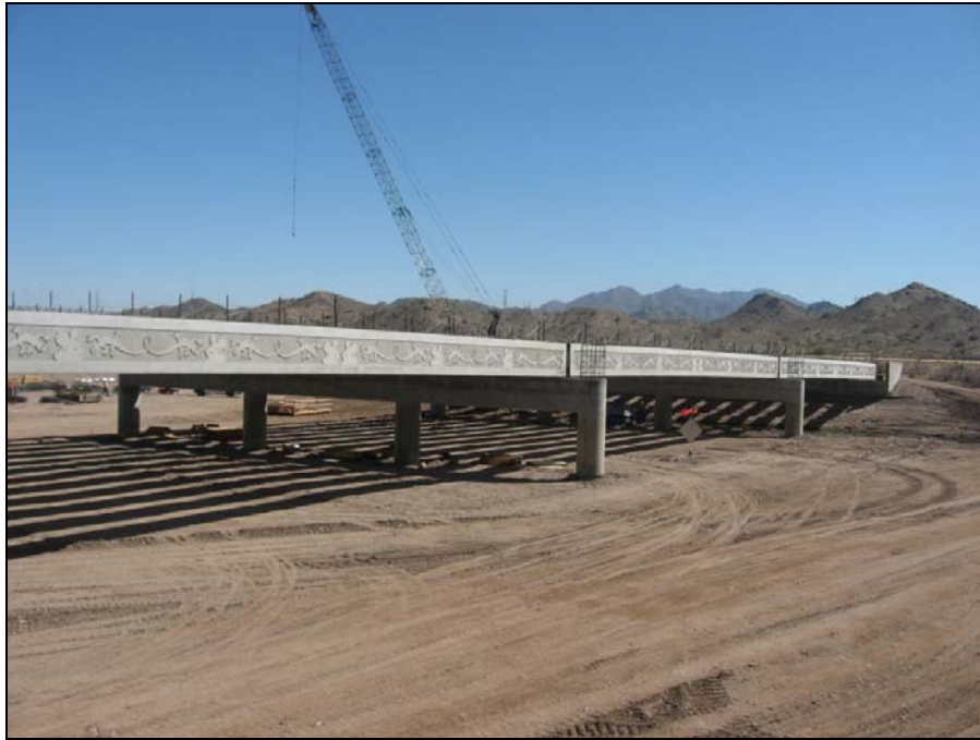
Fig. 2 Girder Placement at Job Site (Before Deck Pour)
