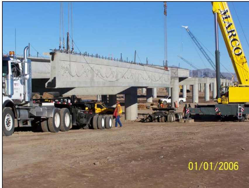
Fig. 7 Unloading Girder at Job Site
