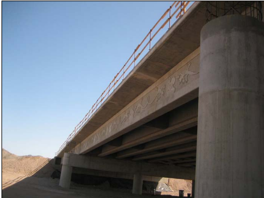
Fig. 3 Exterior Girder at Job Site (After Deck Pour)
