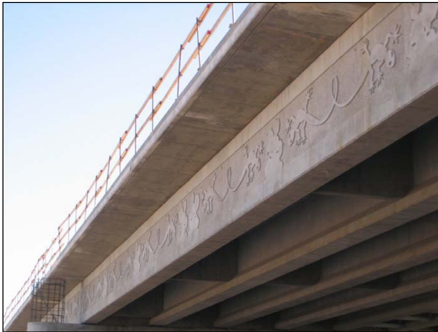
Fig. 6 Girder Elevation with diaphragms
