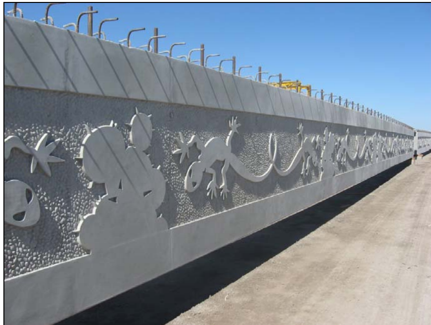
Fig. 1 Exterior Girder at Precast Yard (After Stripping)
