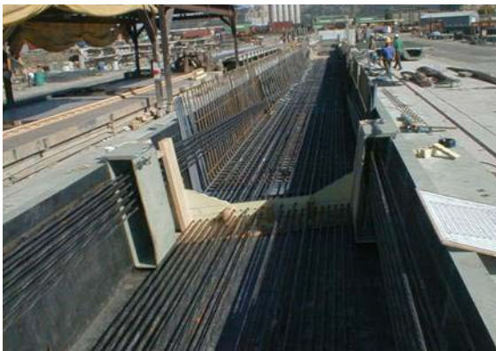
Fig. 6 Outer Steel Form
