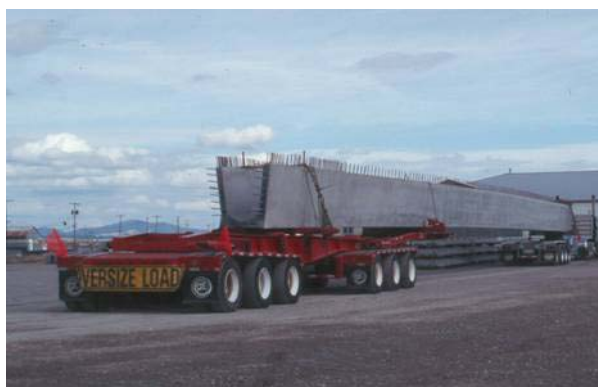
Fig. 5 Hauling of a Tub Girder
