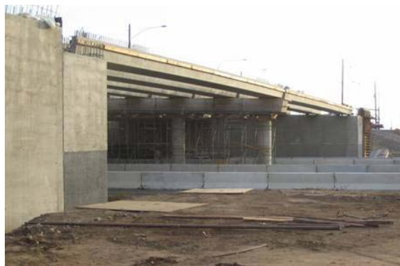
Fig. 10 Tub Girder Bridge Prior to Deck Placement in Yakima, WA
