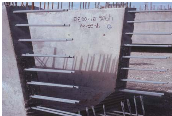
Fig. 3 PC/PS Tub Girder
