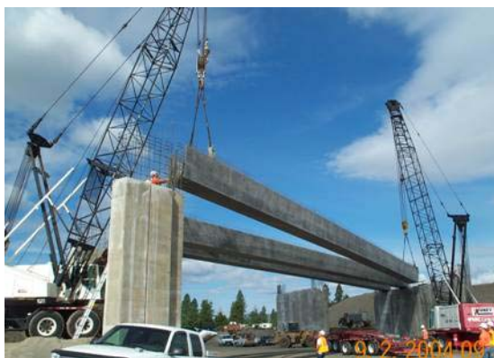
Fig. 9 Tub Girders Being Placed near Spokane, WA
