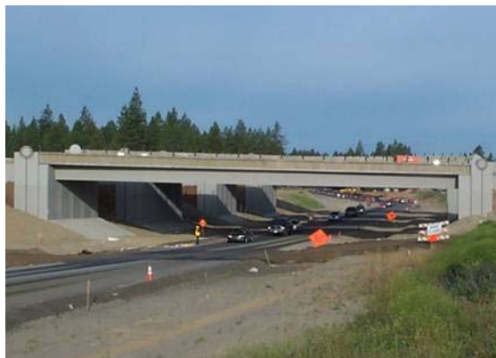
Fig. 8 Tub Girder Bridge near Spokane, WA
