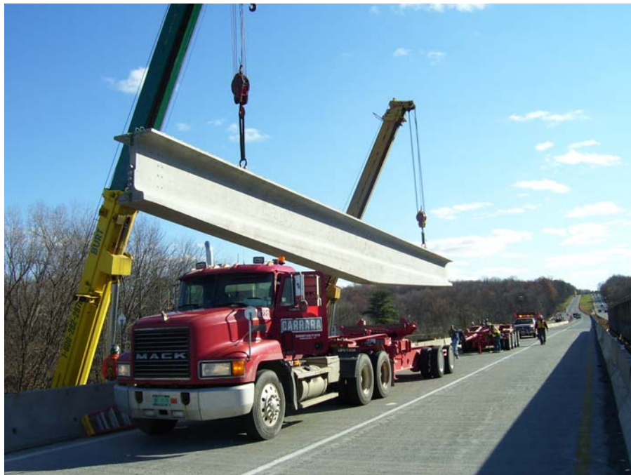
Figure 13 Middle segment being picked up at the quarter points
