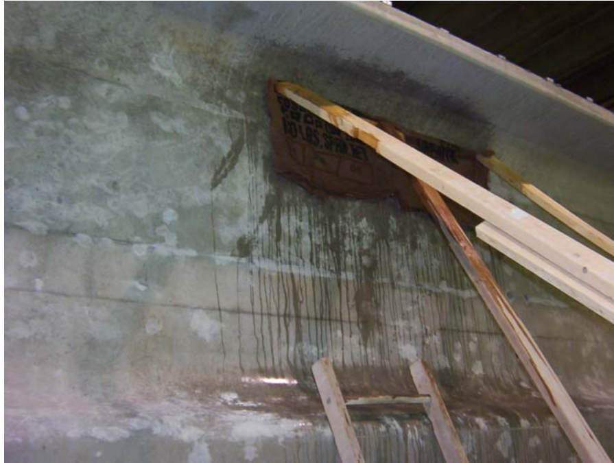
Figure 9- Repair of void in the web
