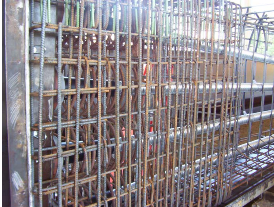
Figure 10 Reinforcing in the anchorage zone
