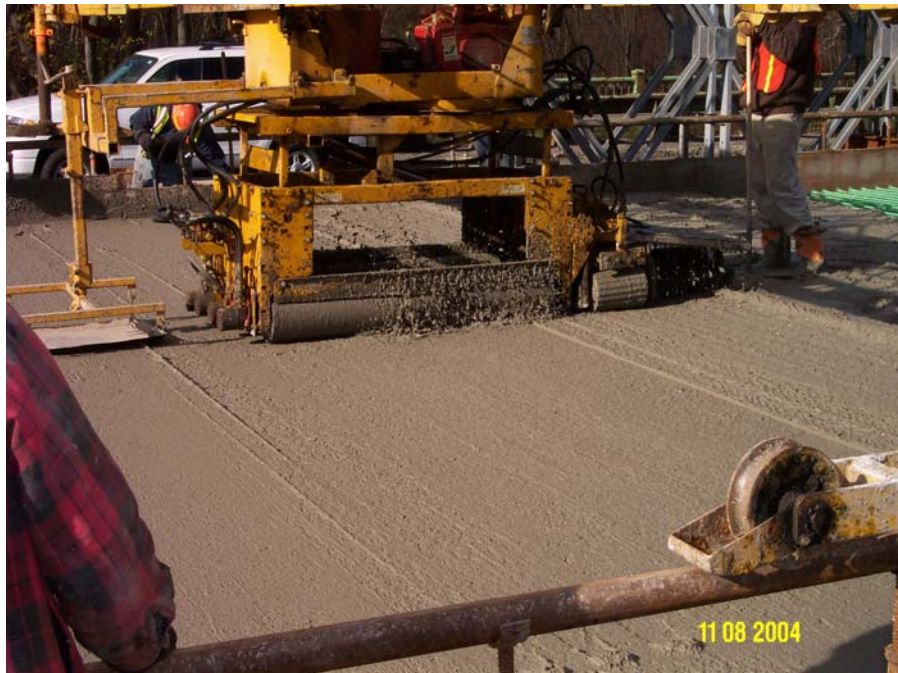
Figure 16 Deck placement operation
