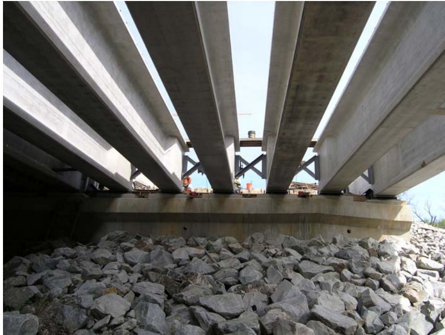
Figure 14 end segments supported at the abutments
