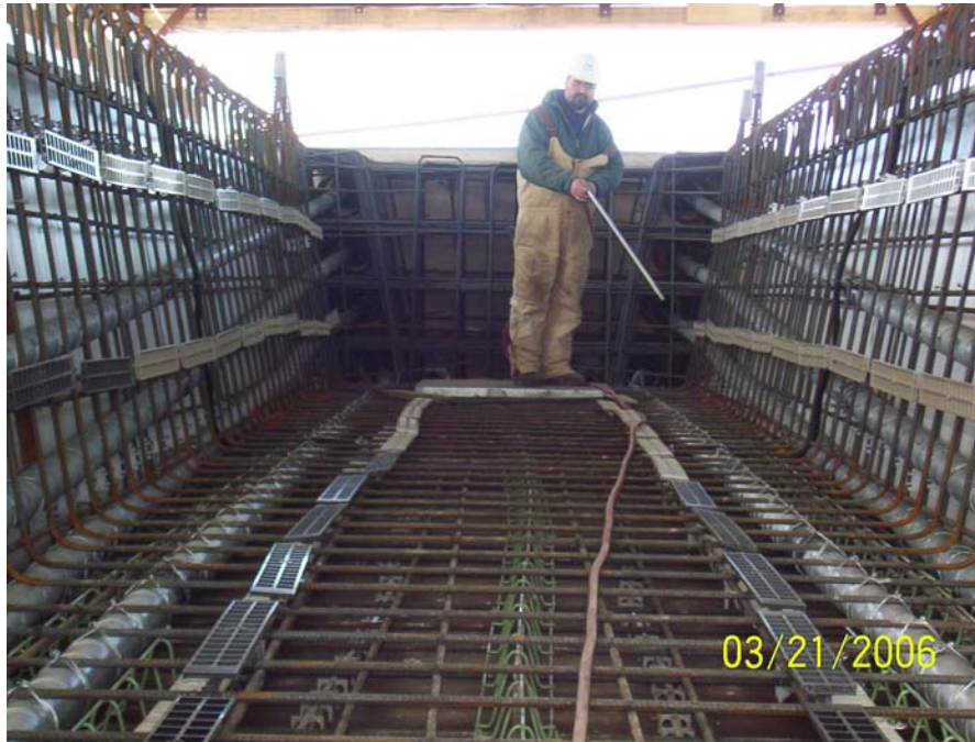
Figure 21 Reinforcement for the bottom and sides of the segment and ready to receive void producing forms
