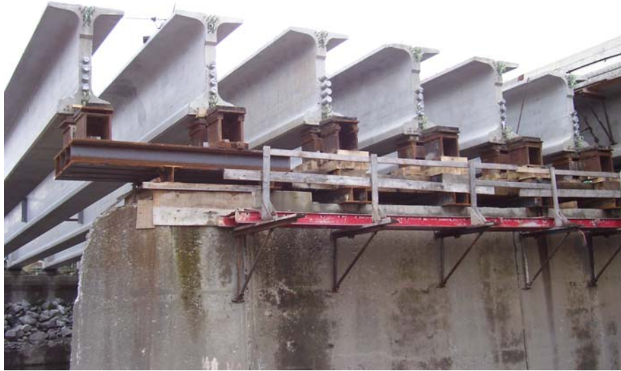
Figure 12 End segments on the temporary support
