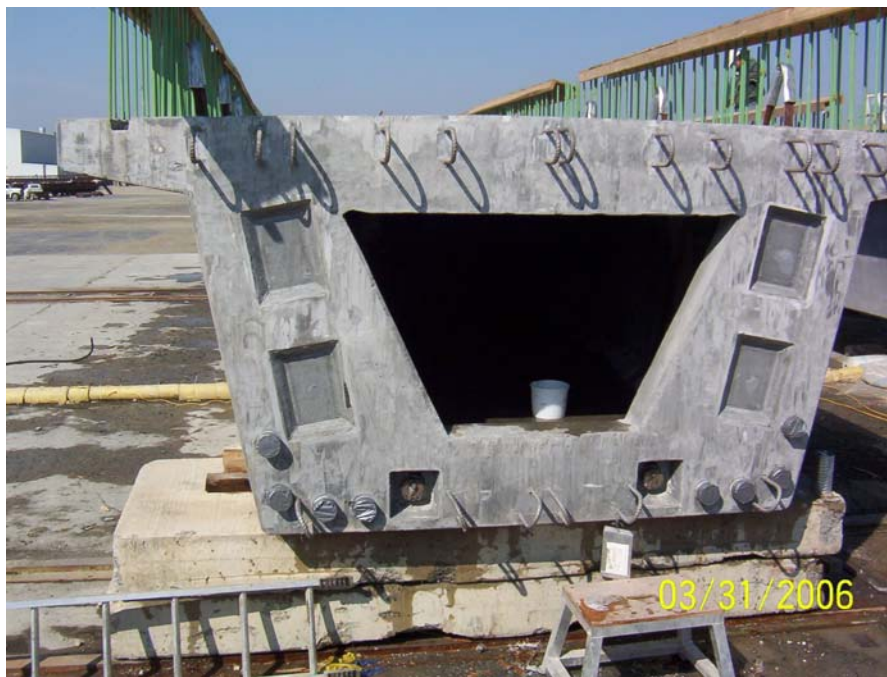
Figure 24 Finished girder segment end view of the splice end
