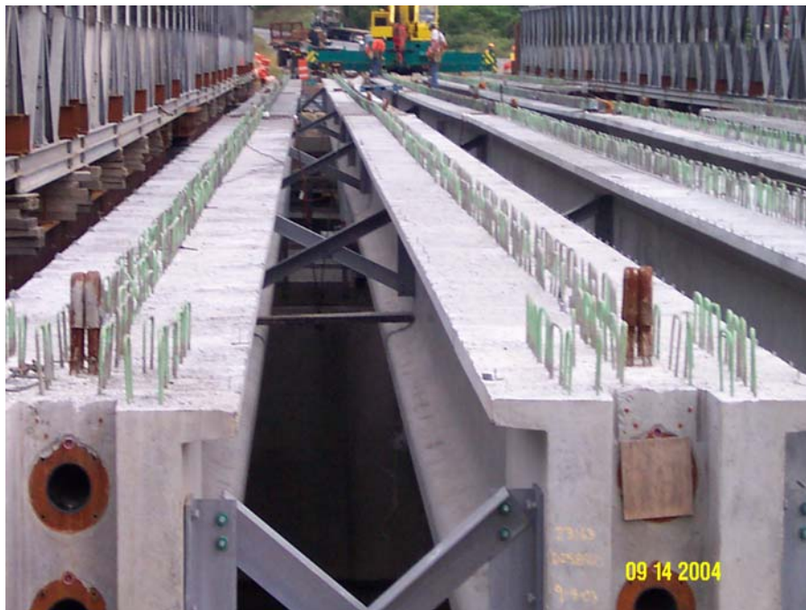
Figure 15 view of girders after installation
