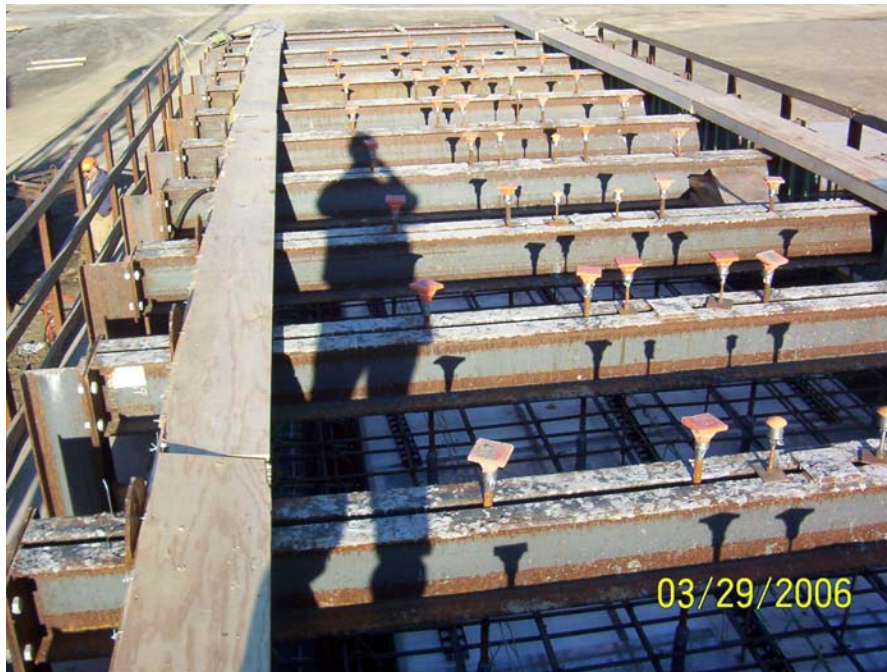
Figure 21 Reinforcement for the bottom and sides of the segment and ready to receive void producing forms
