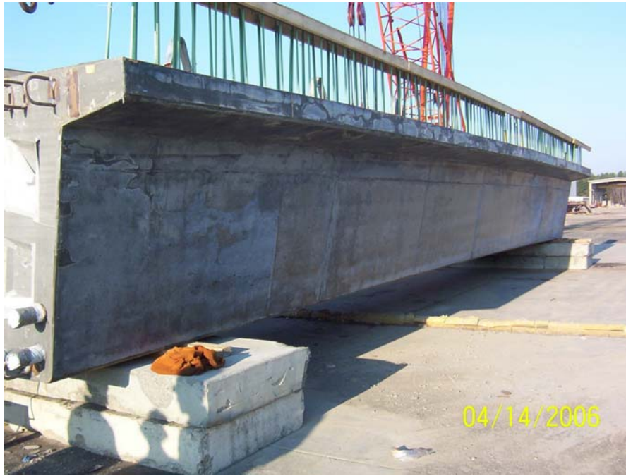
Figure 23 Finished girder segment
