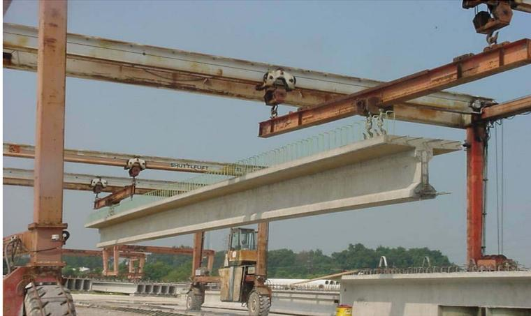
Fig. 10 Finished Deck Girder
