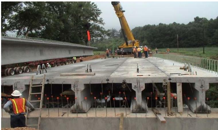
Fig. 11 Installing the Last Deck Girder
