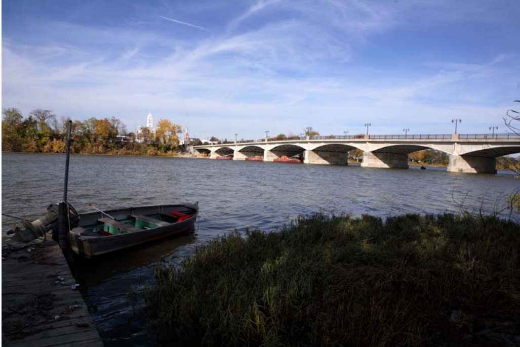
Fig. 9 Completed Bridge Photo by Grand Lubell Photography
