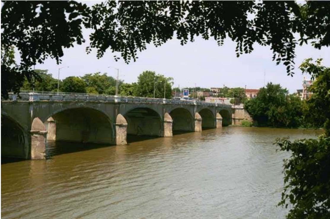
Fig. 1 The 1930 Perry Street Bridge in Napoleon, Ohio before replacement
