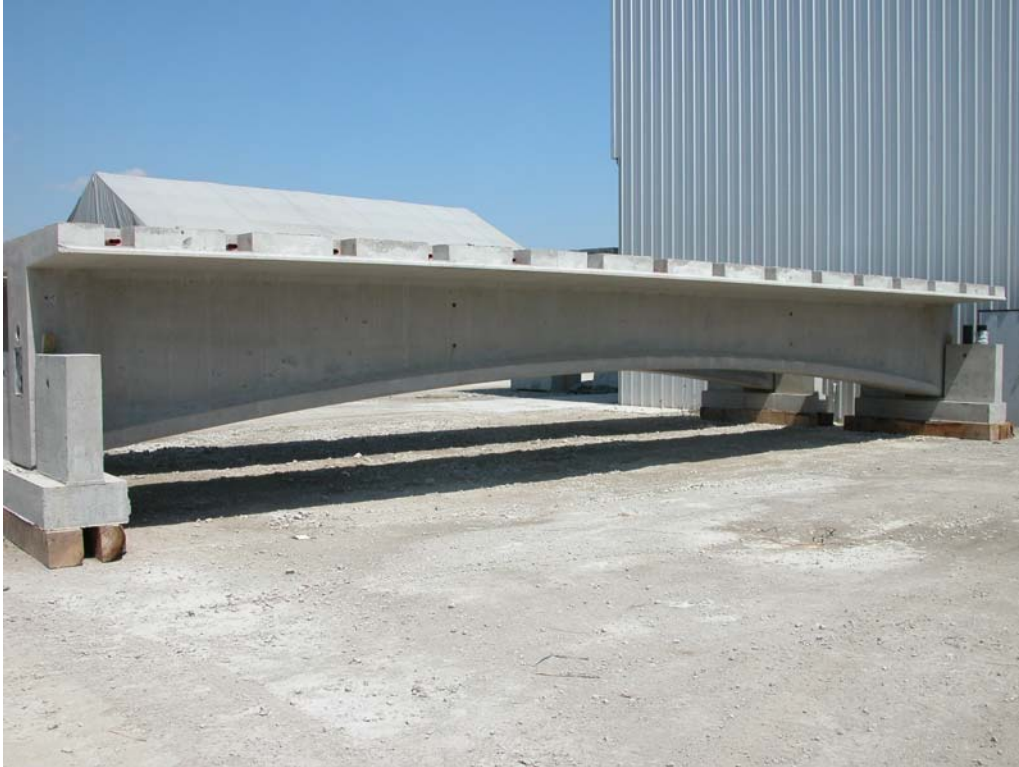
Fig. 6 The mid-span modules had to be supported from tipping over due to the center of gravity being right underneath the top slab.
