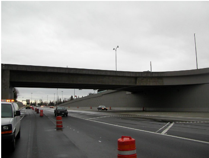
Figure 1 – Southbound I-5 at S. 317 th Street, Looking North
