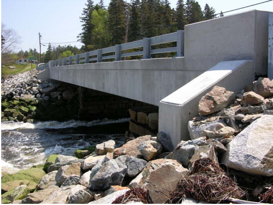
Photo 9: Completed Bridge photo taken 9 months after completion.
