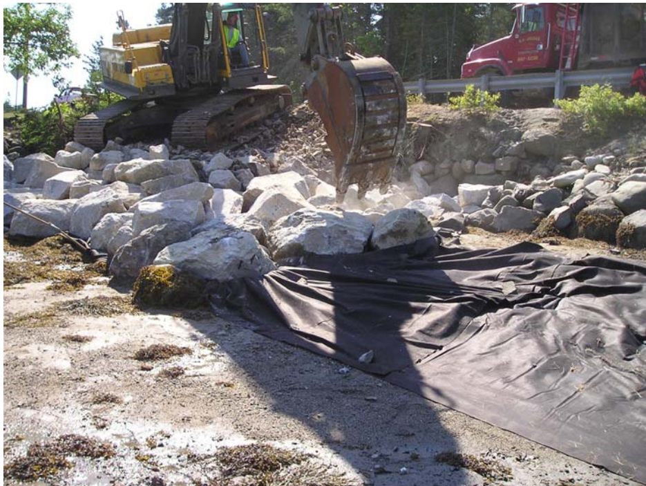
Photo 2: Extensive use of Geotextiles to stabilize Causeway.
