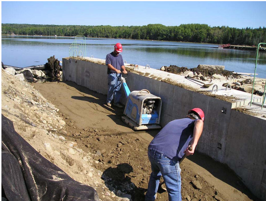
Photo 6: All four Precast Abutment units in place
