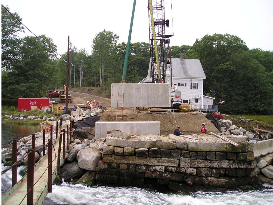
Photo 3: Placement of Center Precast Abutment units.
