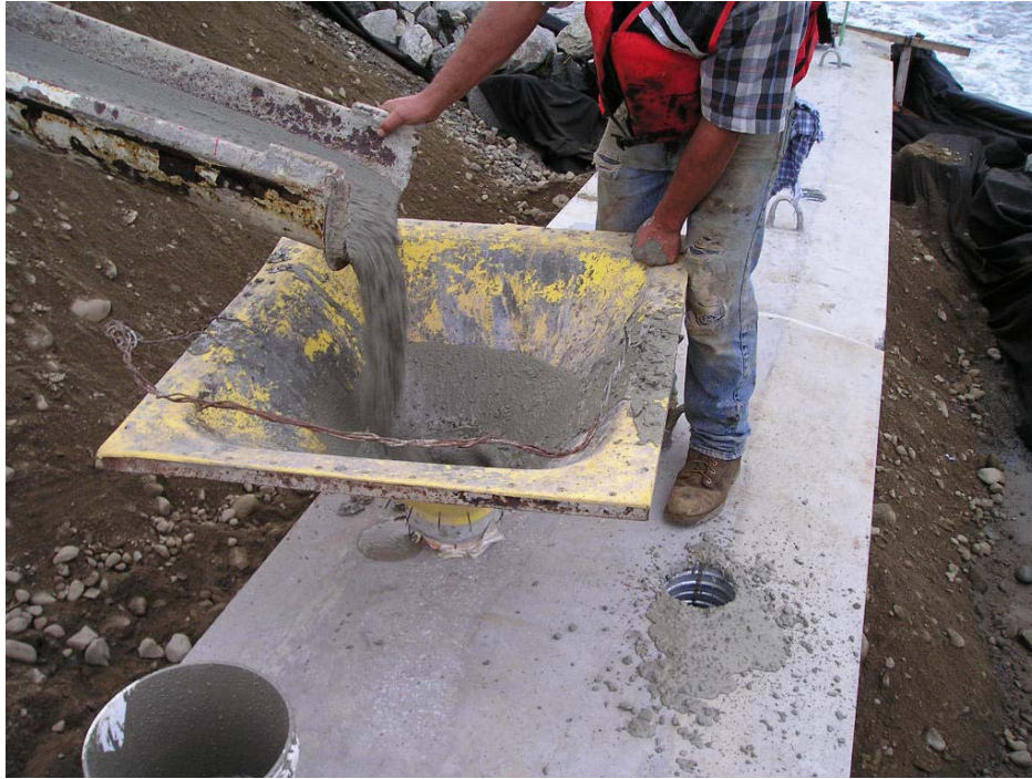
Photo 5: Self-Consolidating Concrete poured into the voids.
