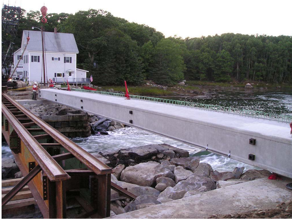
Photo 7: Launching Beam and first Precast Box beam in place.
