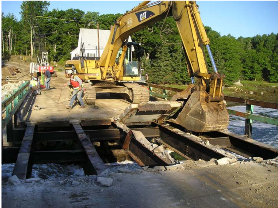
Photo 1: Removal of Existing Steel Girder Bridge.
