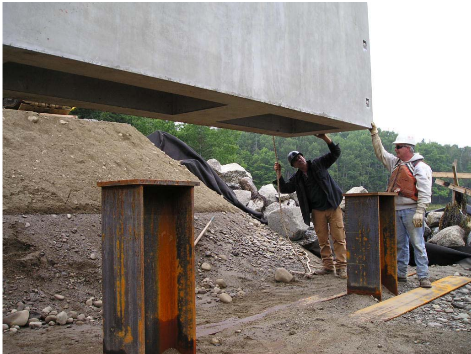
Photo 4: Precast Abutment voids being aligned with Pile tips.
