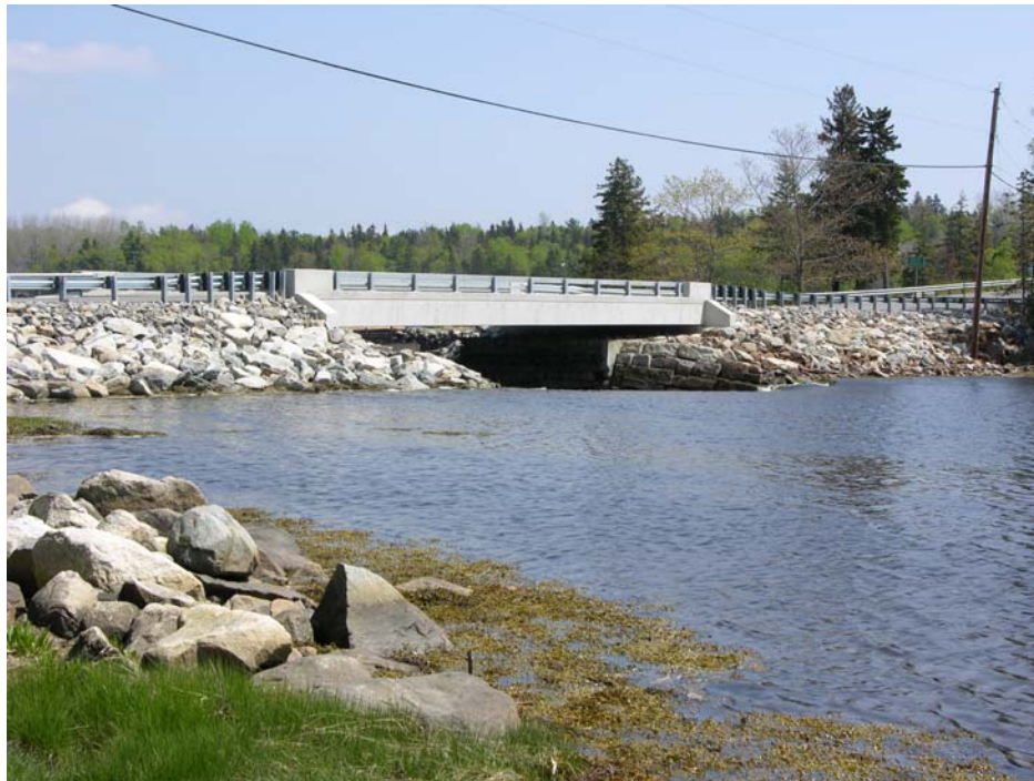
Photo 8: Completed Bridge showing causeways.
