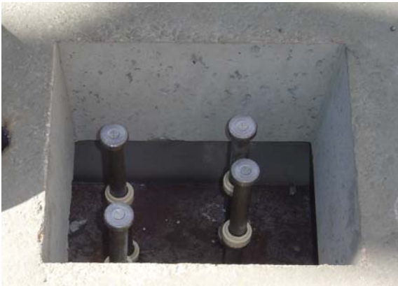
Figure 3: Typical Block-Out with Headed Anchor Studs
