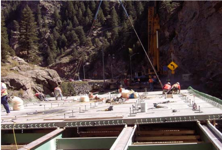
Figure 7: Deck panels being set and adjusted using elevation screws
