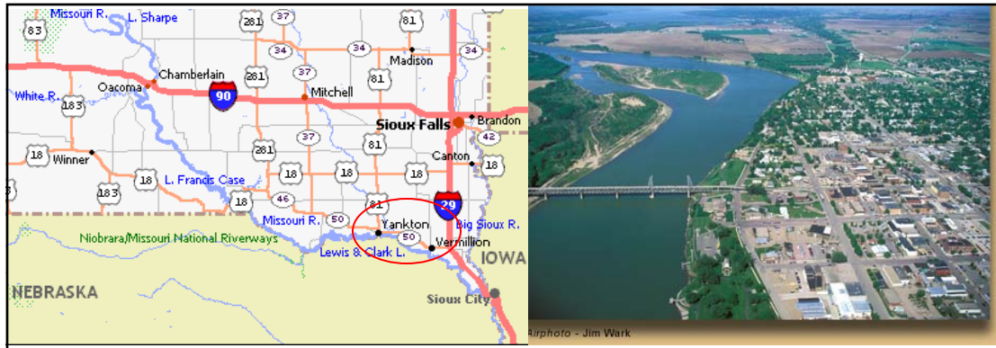
Fig. 1 Location and Photograph of Current Yankton Bridge
