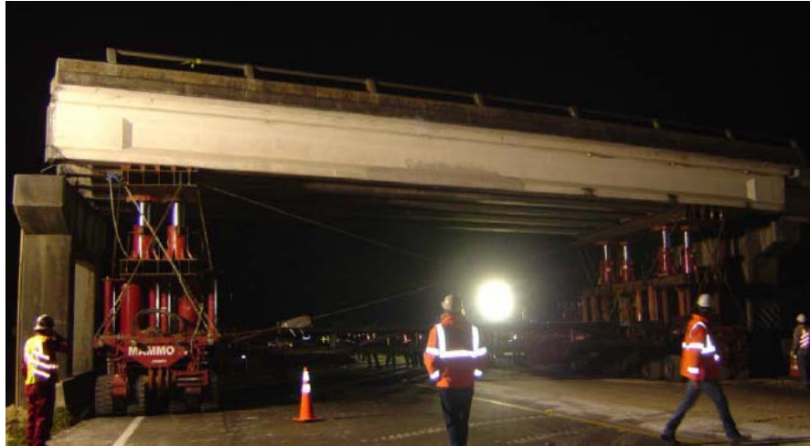
Fig. 3 Removal of Existing Span over I-4 East, Florida
