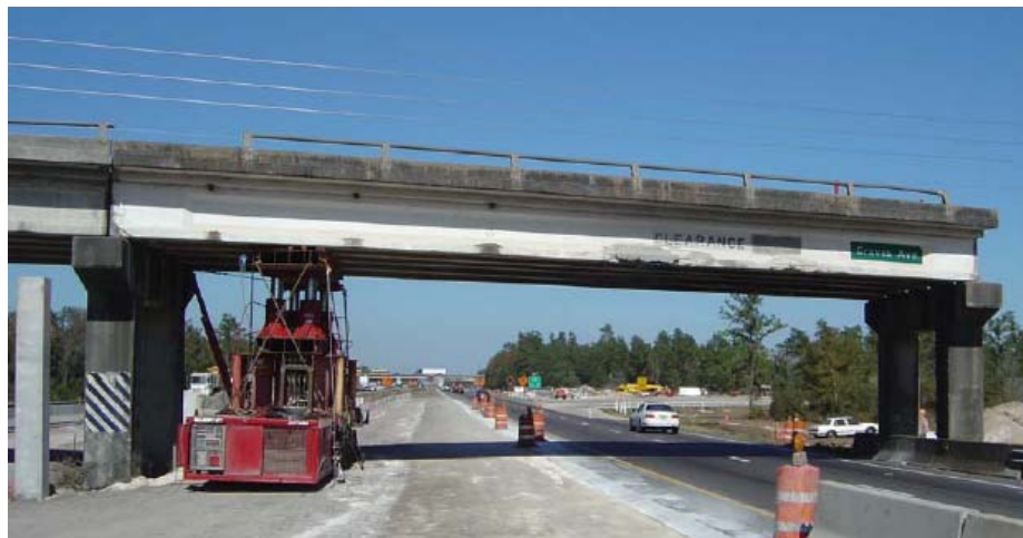
Fig. 2 Pre-positioned SPMT Unit at Existing Span over I-4 East, Florida
