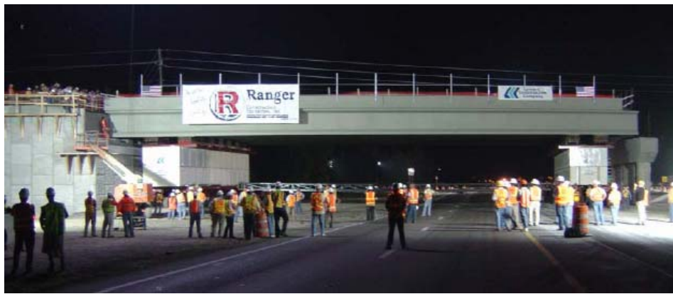
Fig. 4 Installation of Graves Avenue Span over I-4 West, Florida
