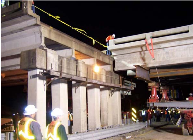
Fig. 6 Installation of New I-10 East Span, Louisiana
