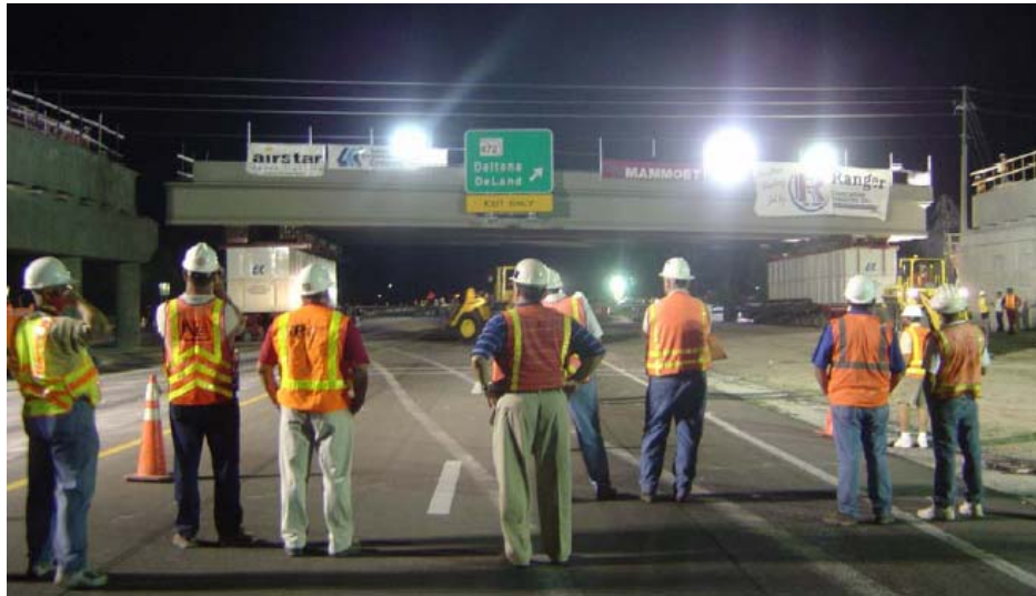
Fig. 5 Installation of Graves Avenue Span over I-4 East, Florida
