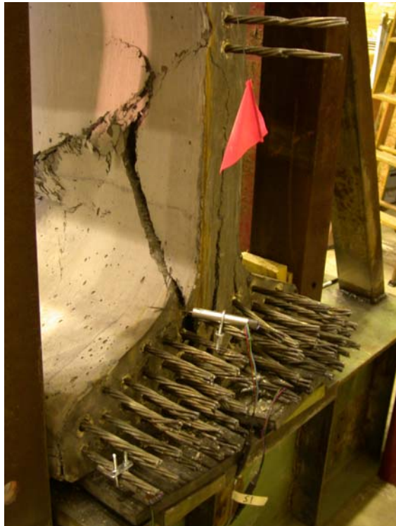
Figure 16. Split beam end.
